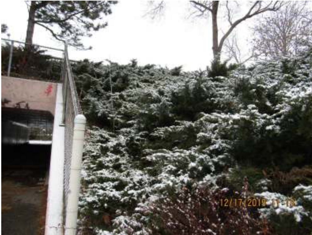
37 South east embankment
