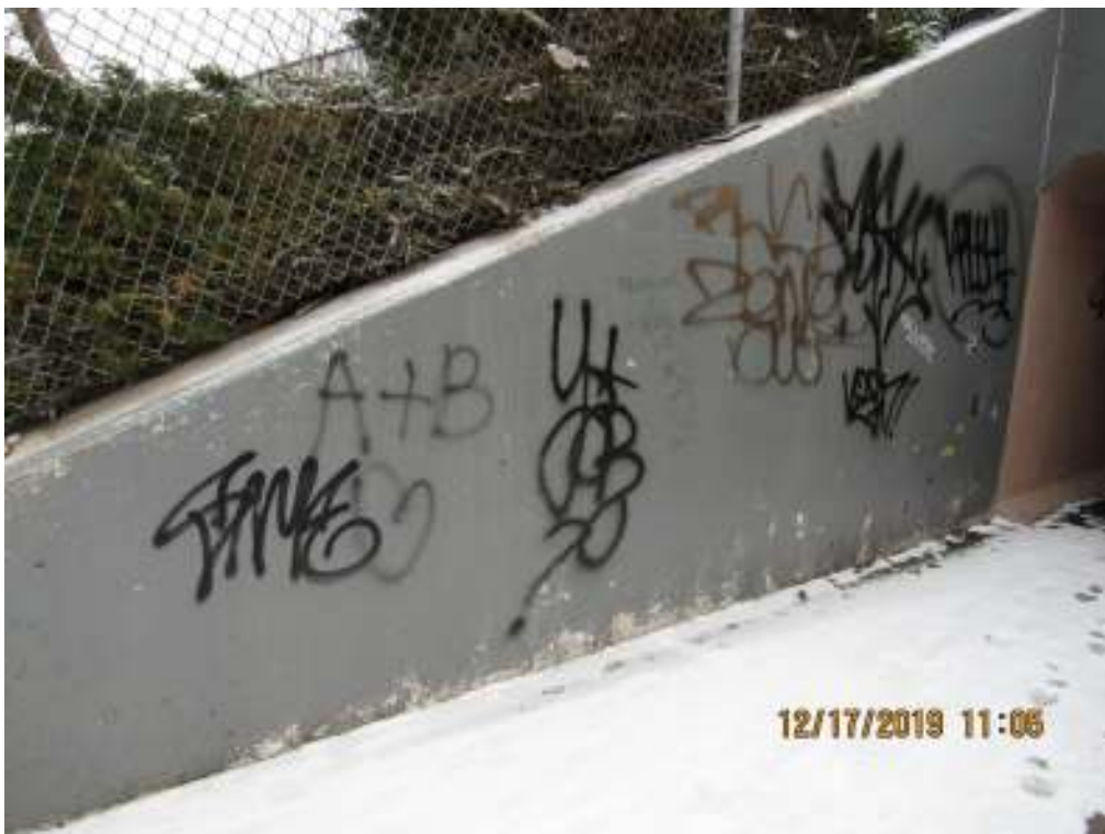
16 North east retaining wall
