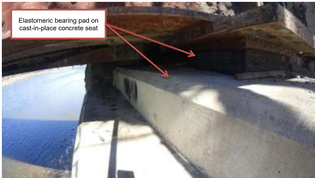
Figure 2: Replaced abutment bearing on Bridge 143
