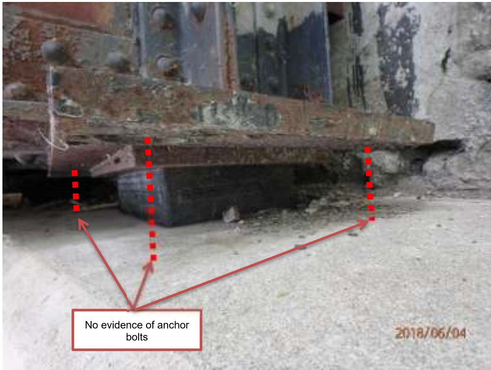
Photograph 5: East abutment, south bearing
