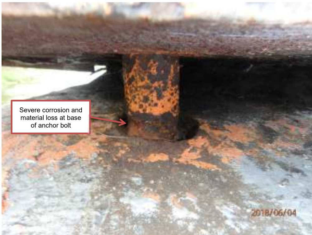
Photograph 12: East pier, anchor bolt at location A25
