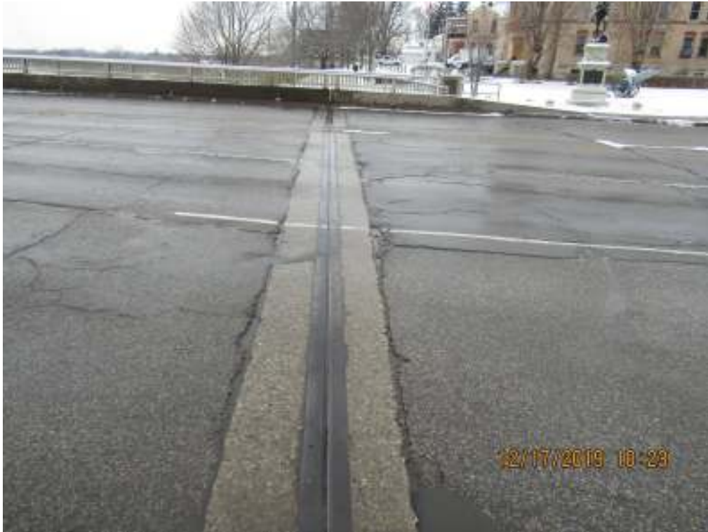
07 East expansion joint
