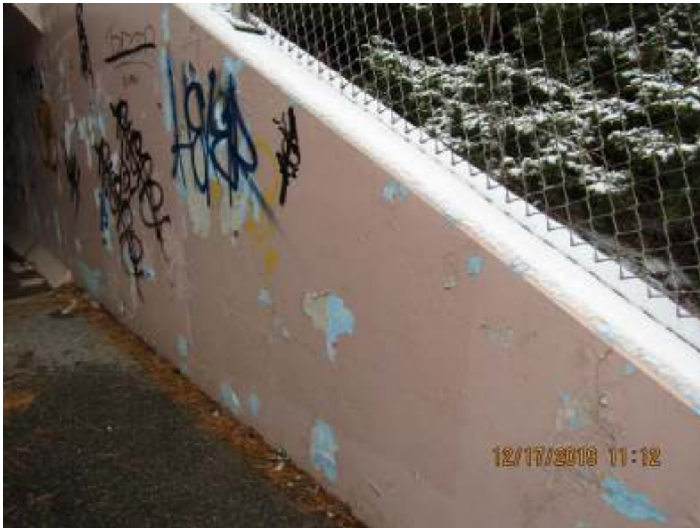
18 South east retaining wall
