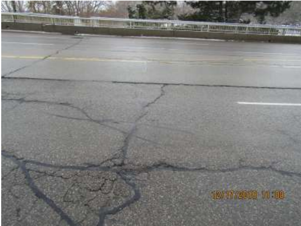
03 Roadway at top of culvert looking south
