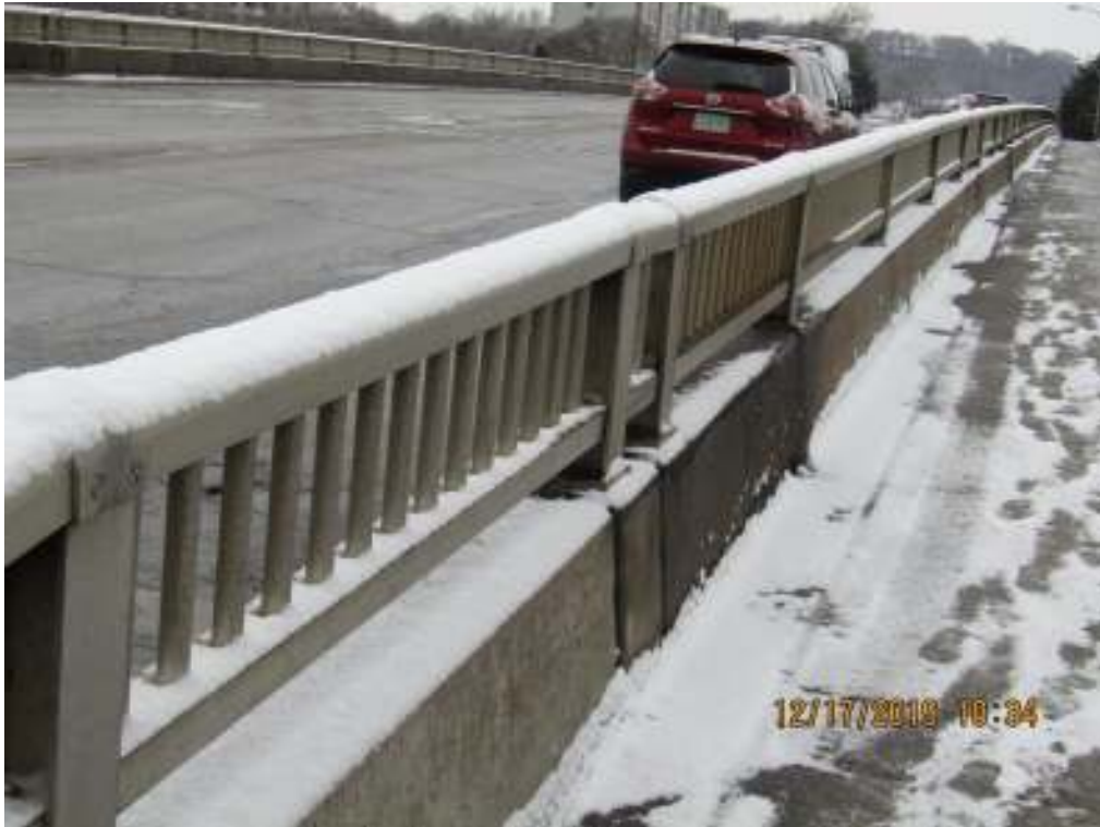
57 North barrier wall
