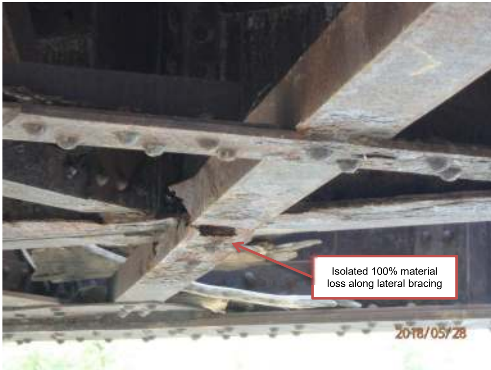
Photograph G13: East span, underside
