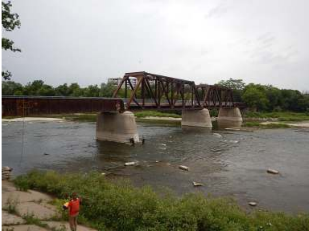
Photograph G1: North elevation
