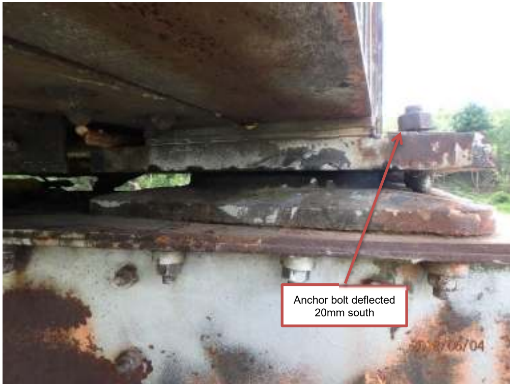
Photograph 11: Center pier, Span #2, north bearing
