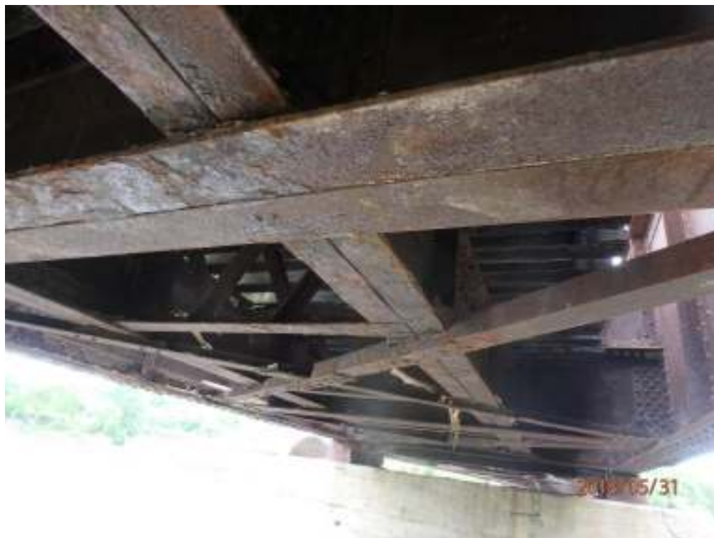
Photograph G16: West span underside
