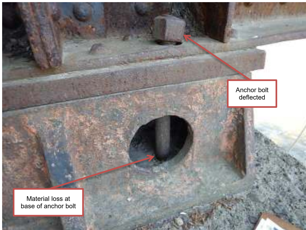
Photograph G4: East abutment, north bearing anchor bolt
