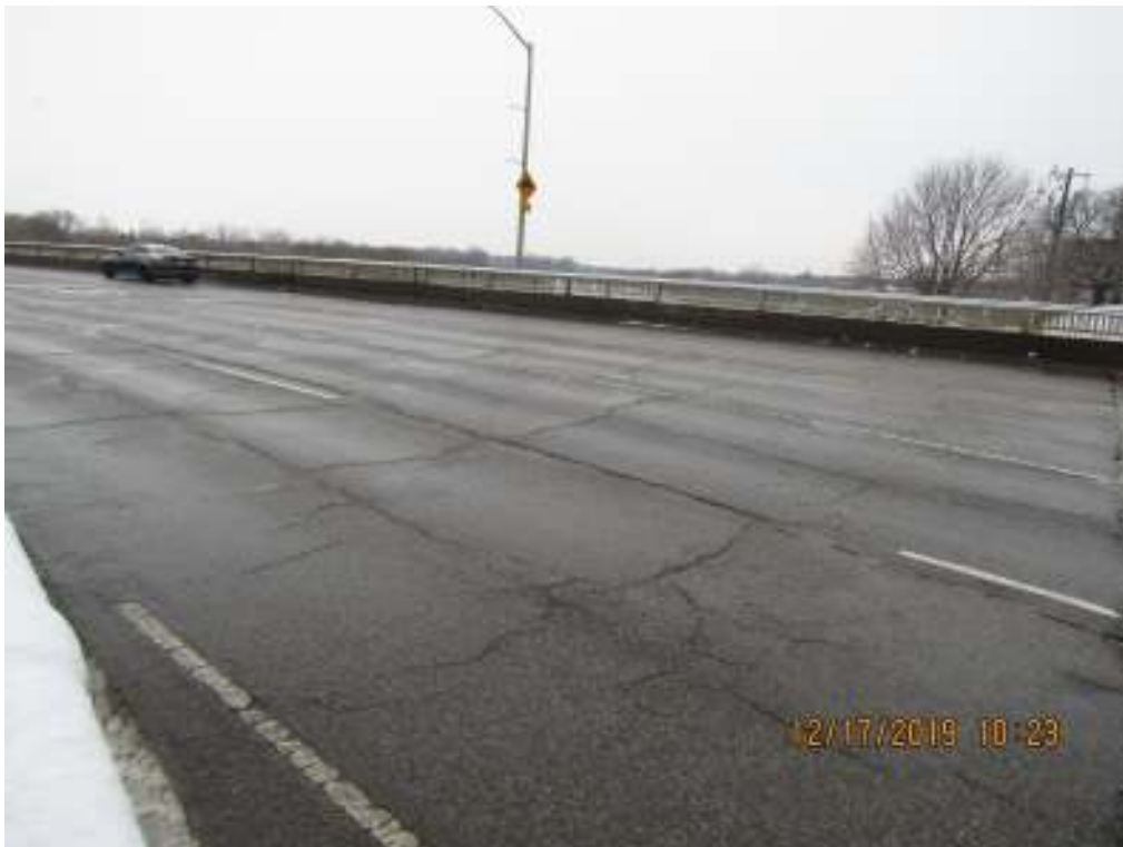
04 Deck, looking west
