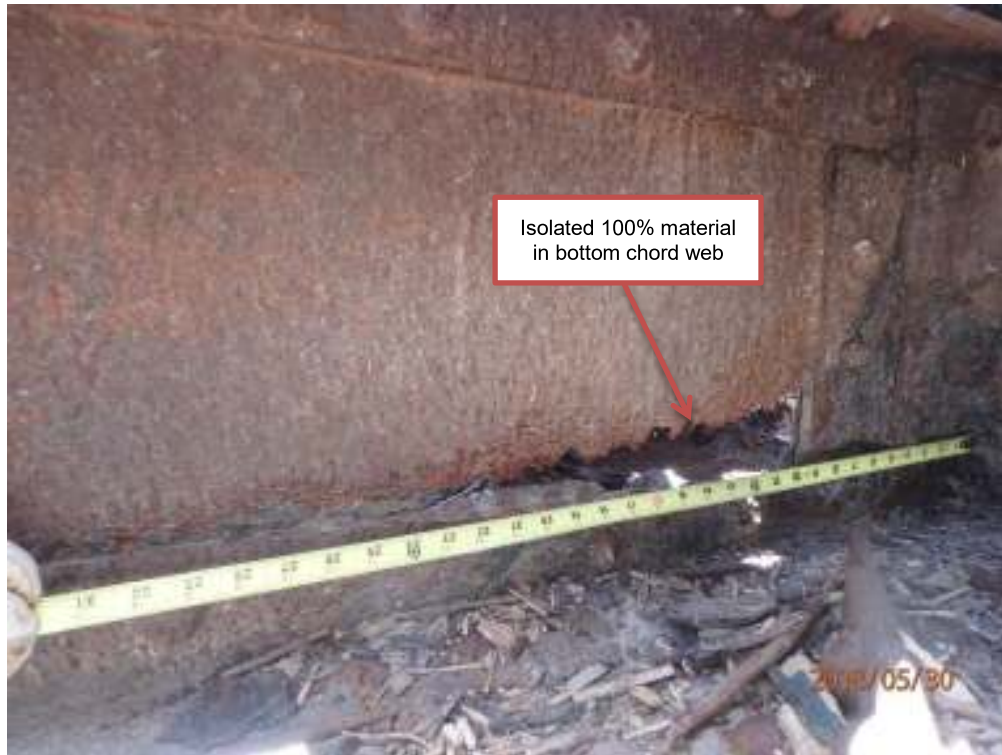
Photograph T9: West truss, bottom chord
