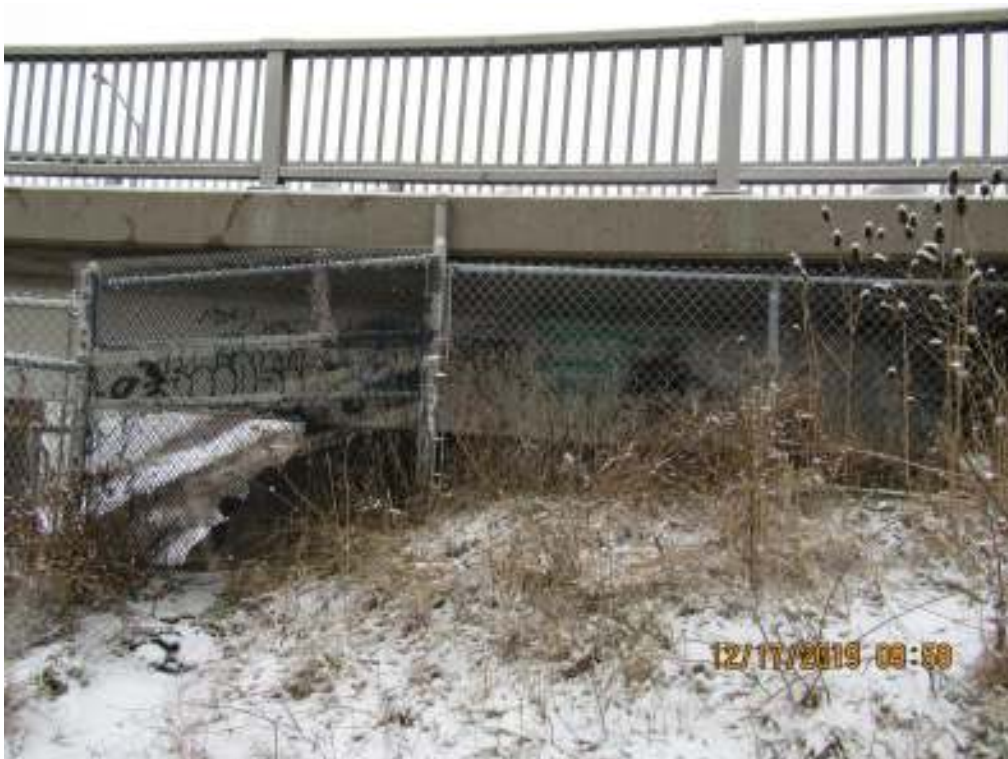
80 Chain link fence at south side
