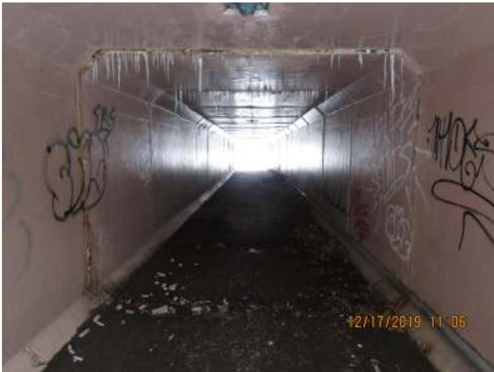
06 Barrel, looking south
