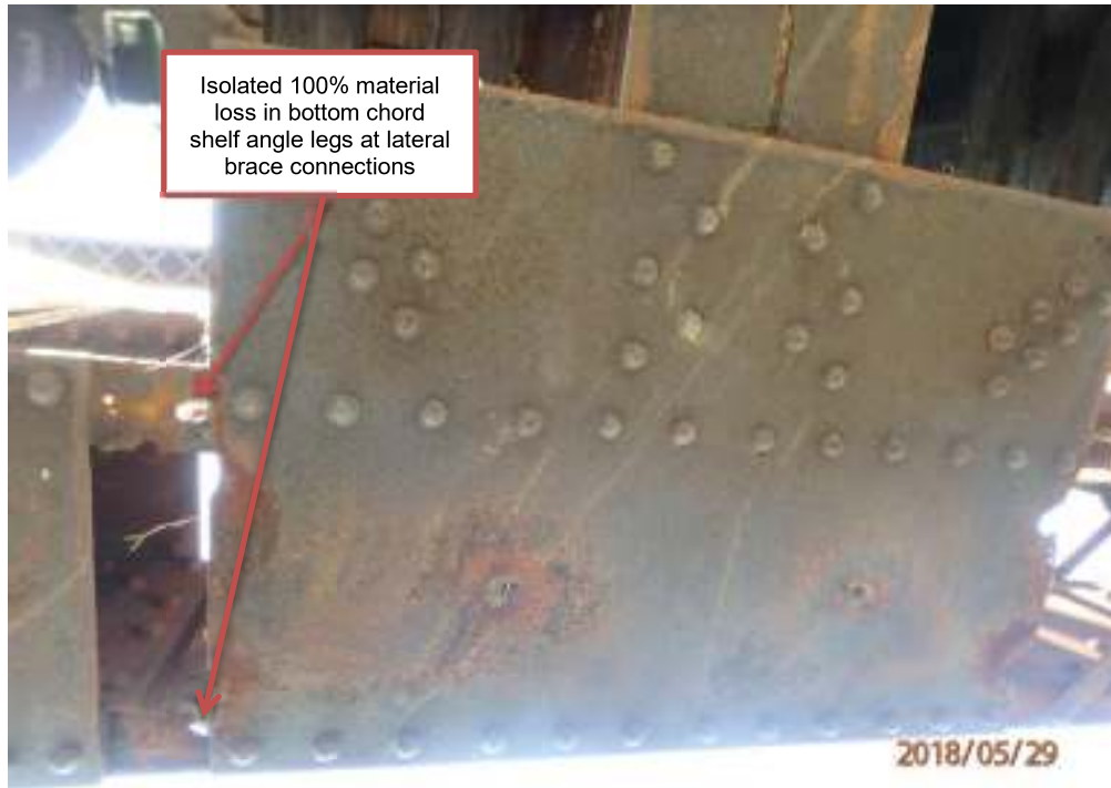
Photograph T5: East truss, bottom chord at lateral brace connection
