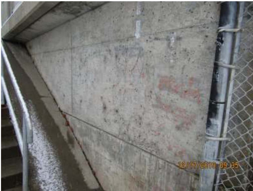
38 North east wingwall
