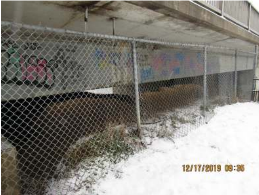
81 Chain link fence at north east end
