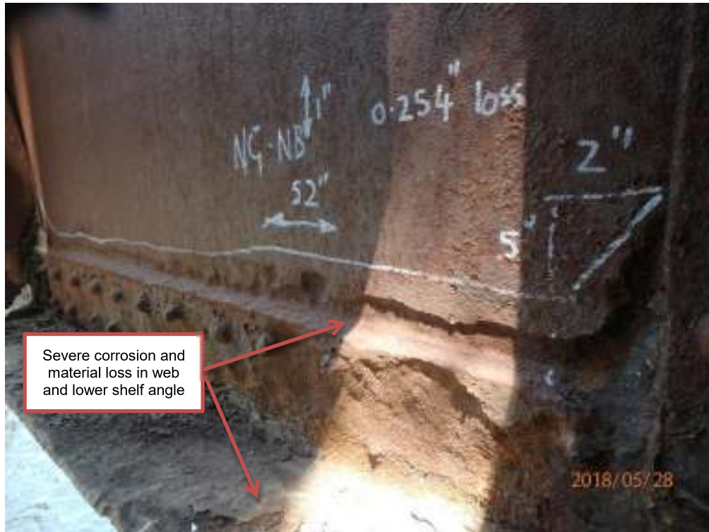
Photograph G8: East span, north girder interior
