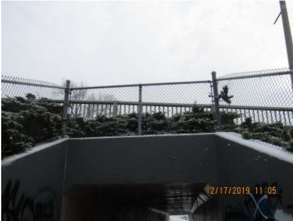
31 Chain link fence on north face
