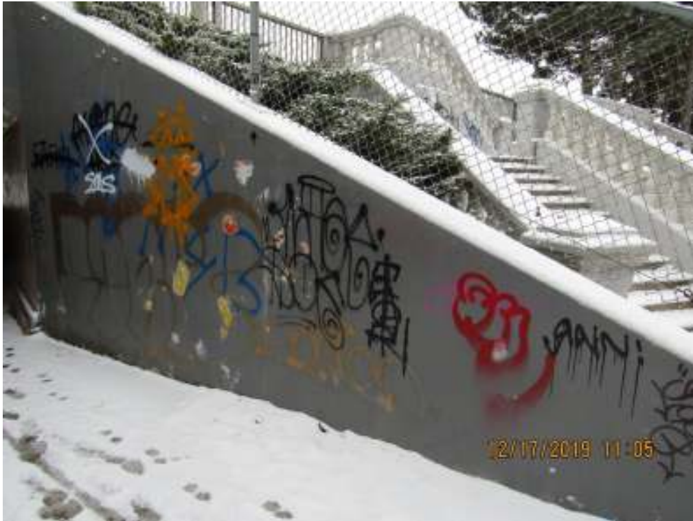
17 North west retaining wall
