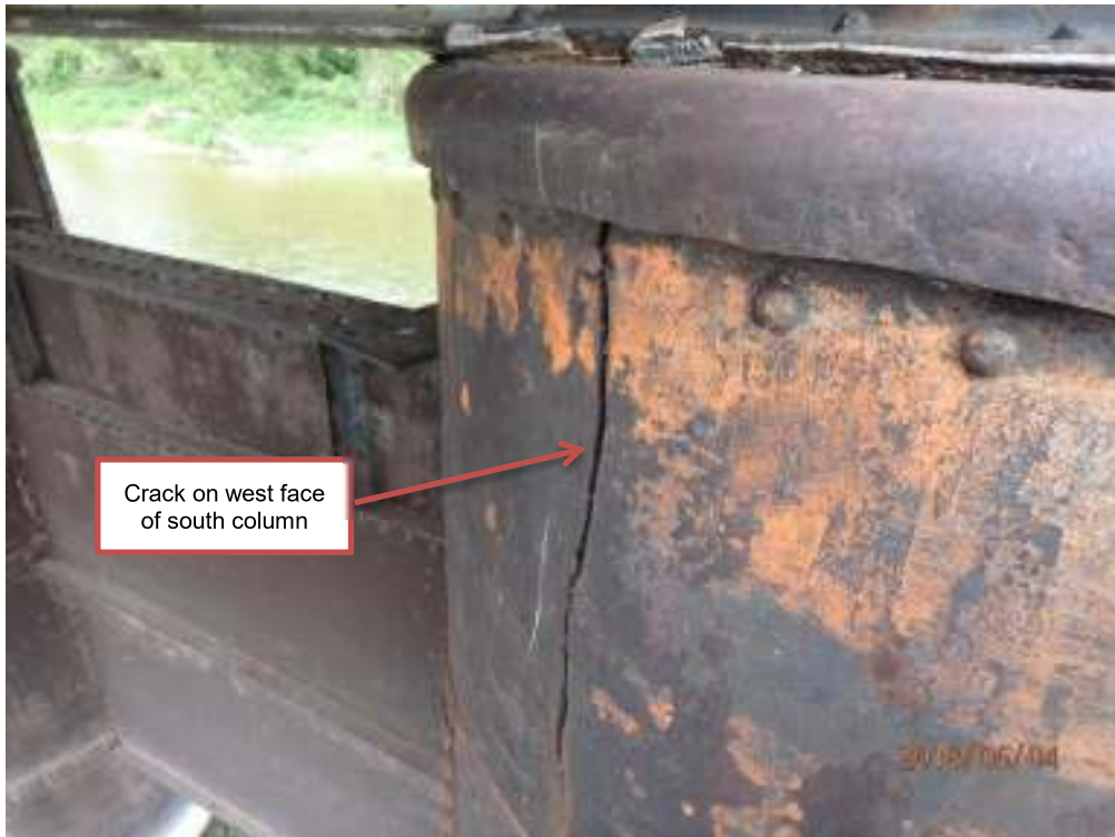
Photograph 10: East pier, south steel column
