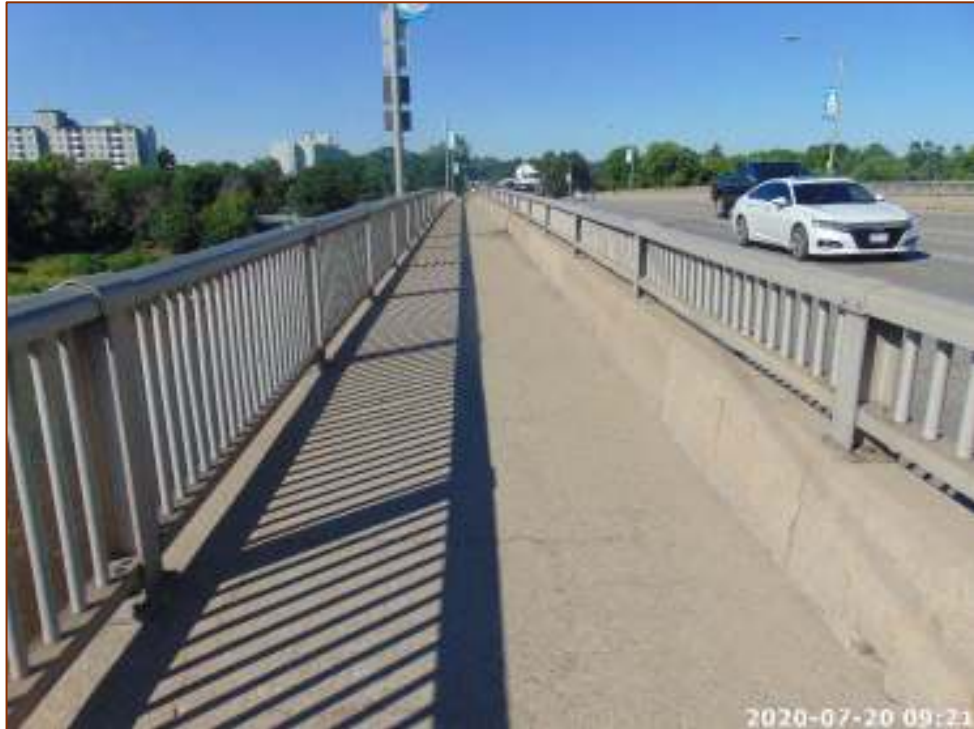
Photo 5 – South Sidewalk, Looking West
