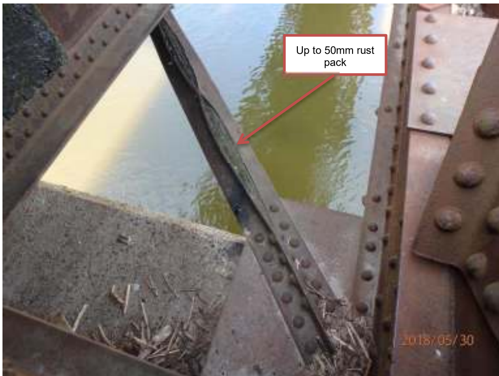
Photograph T14: West truss, lateral bracing
