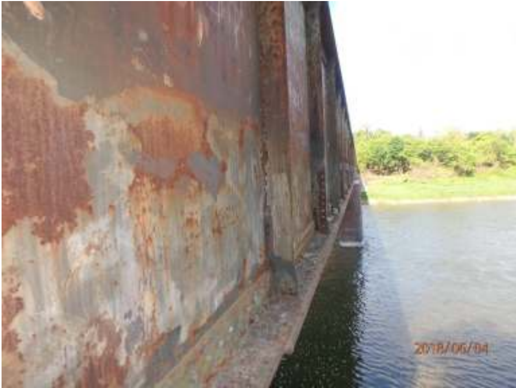
Photograph 15: North plate girder, looking west
