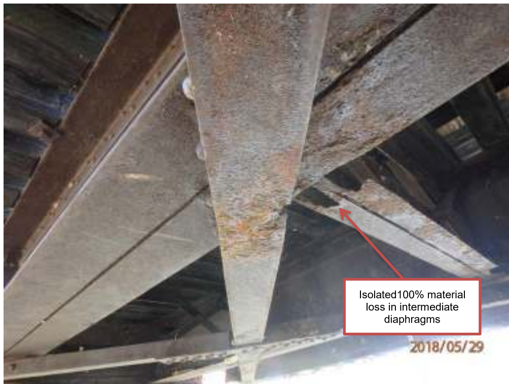
Photograph T12: East truss, underside
