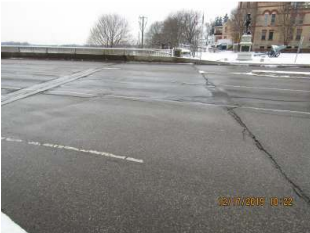
66 East approach slab
