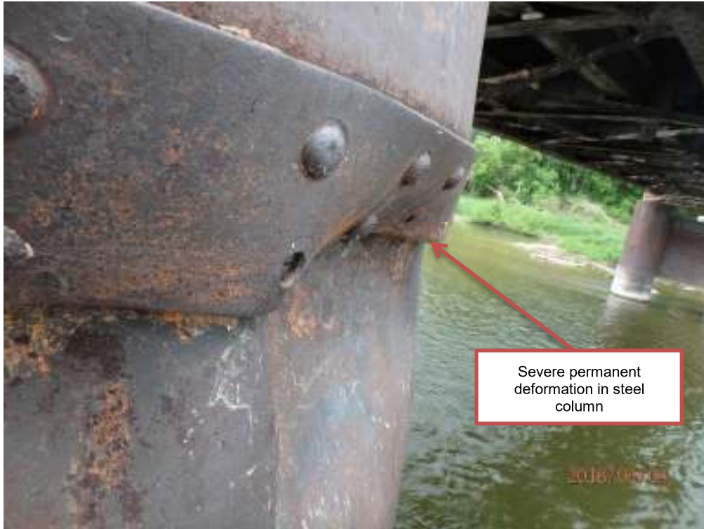
Photograph 9: East pier, north steel column (north face)
