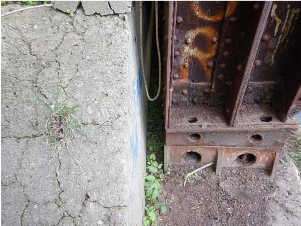
Photograph G5: West abutment, south bearing
