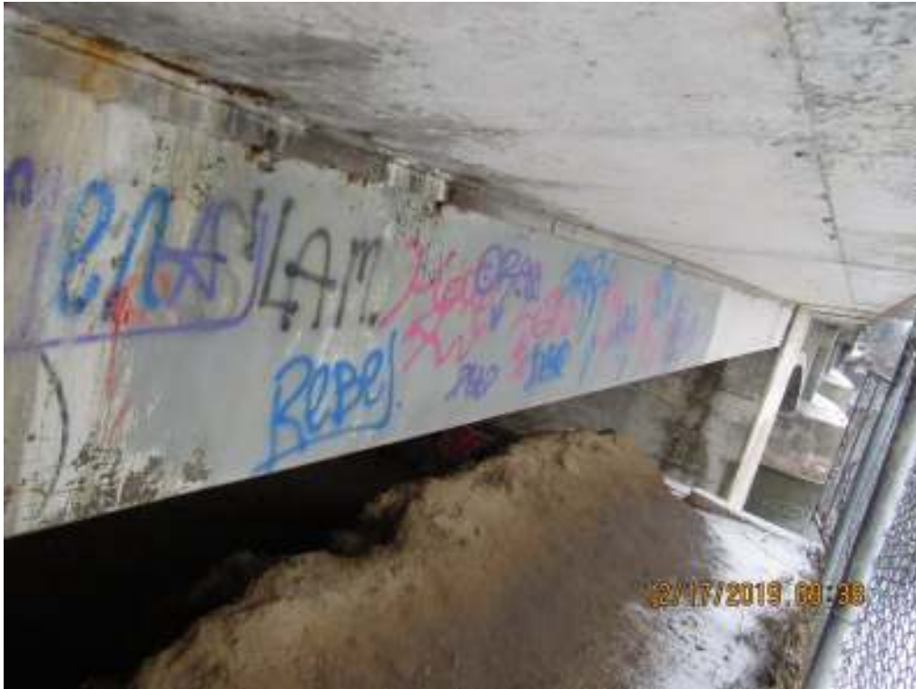
23 North exterior girder
