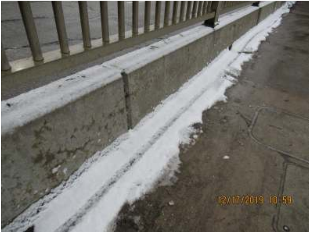
23 North barrier wall
