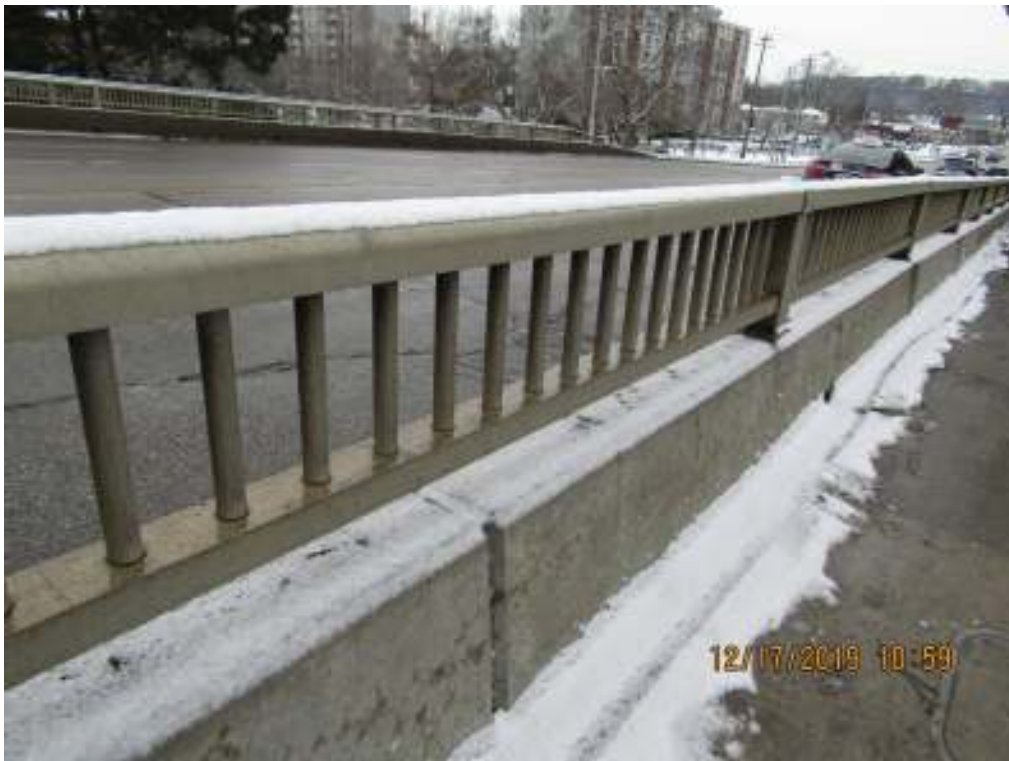
26 North barrier railing
