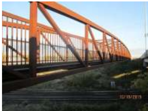
Figure 2: Prefabricated steel truss superstructure (Structure 152)
