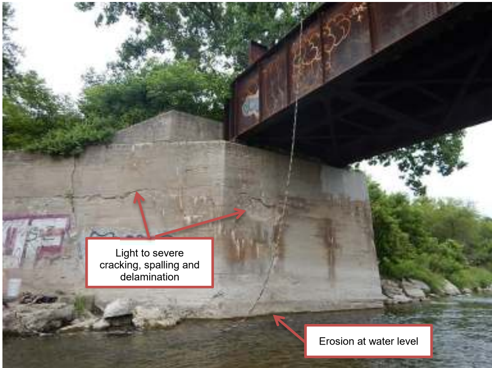
Photograph G2: East Abutment
