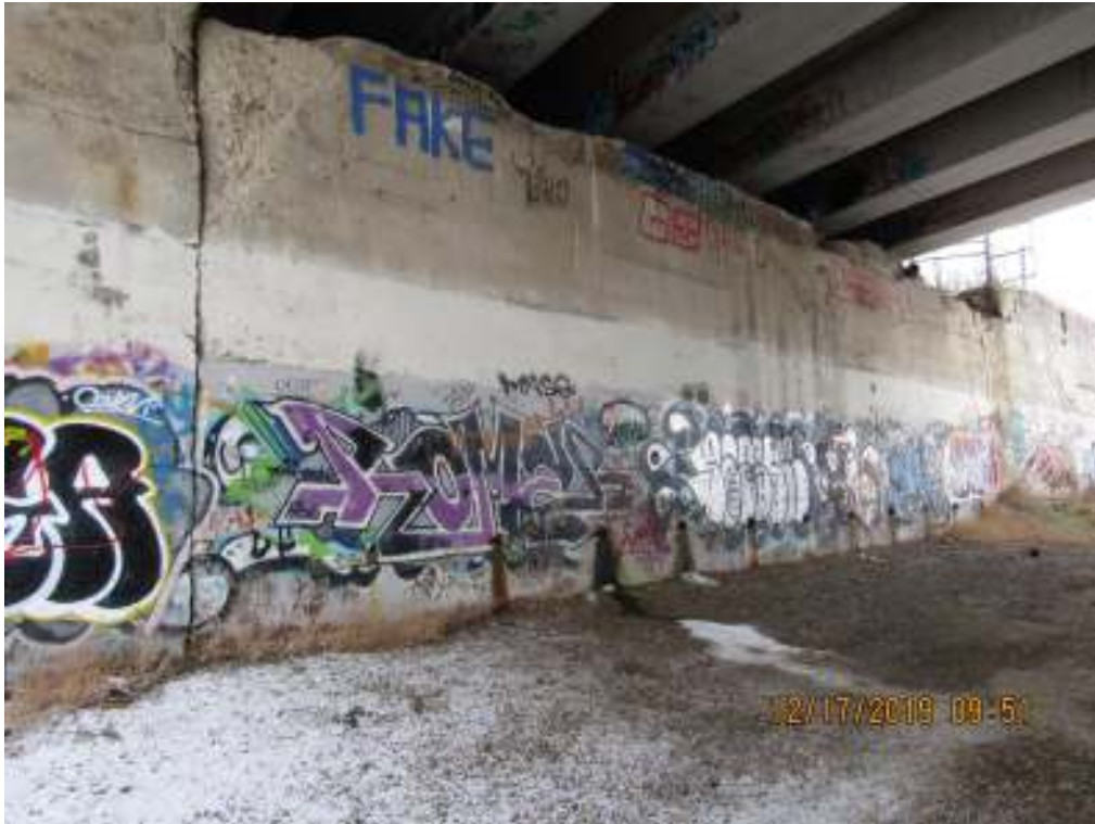
45 East Retaining wall section under bridge
