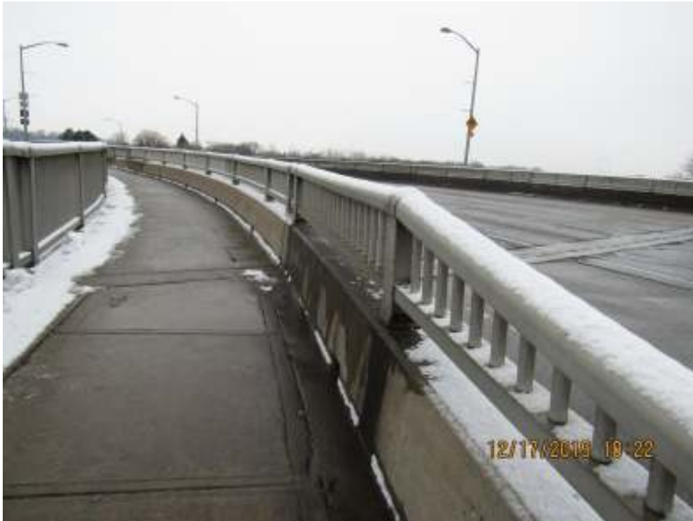
59 South barrier railing system
