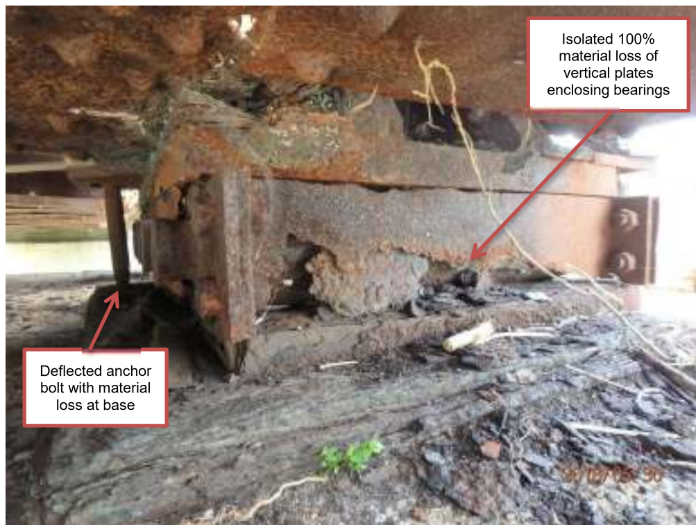
Photograph T4: West pier, north roller bearing
