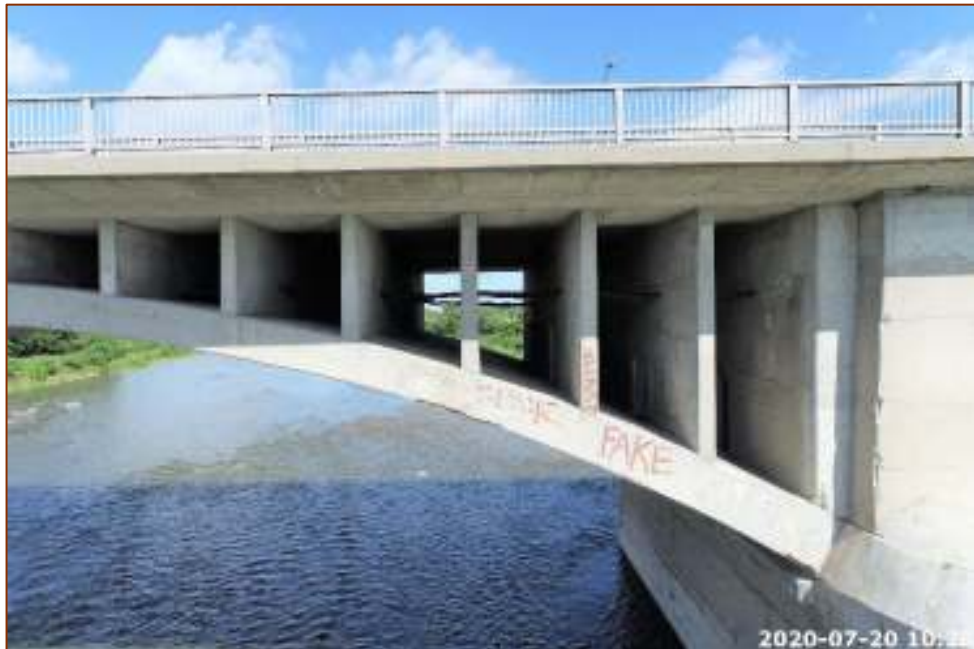
Photo 34 - Centre Span, South Face of Bottom Chord, Spalls & Delaminations
