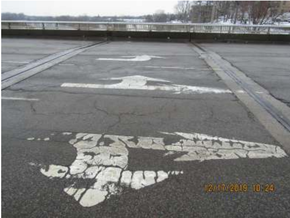
67 West approach slab
