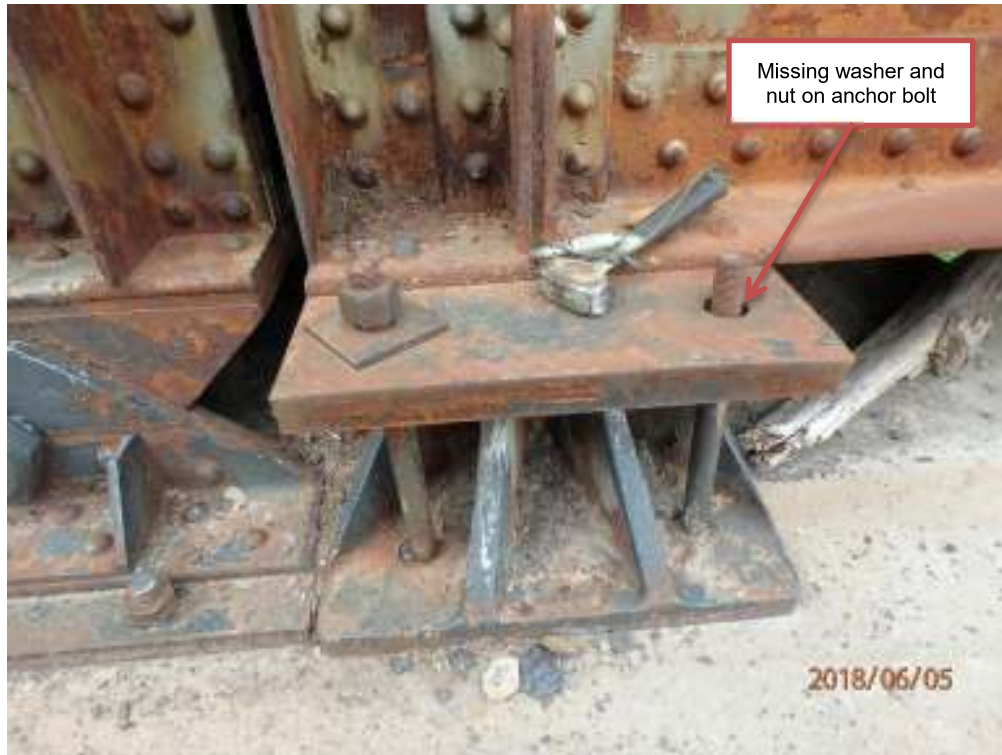
Photograph 13: West pier, bearing at location D9
