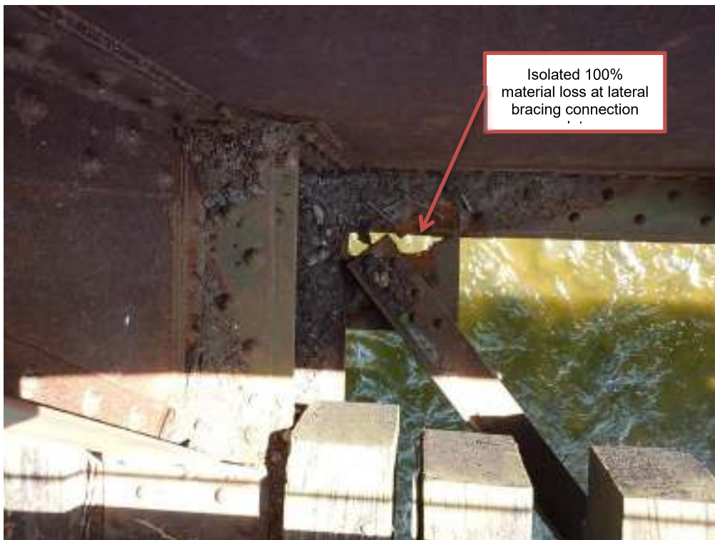
Photograph G14: East span, typical lateral bracing connection plate
