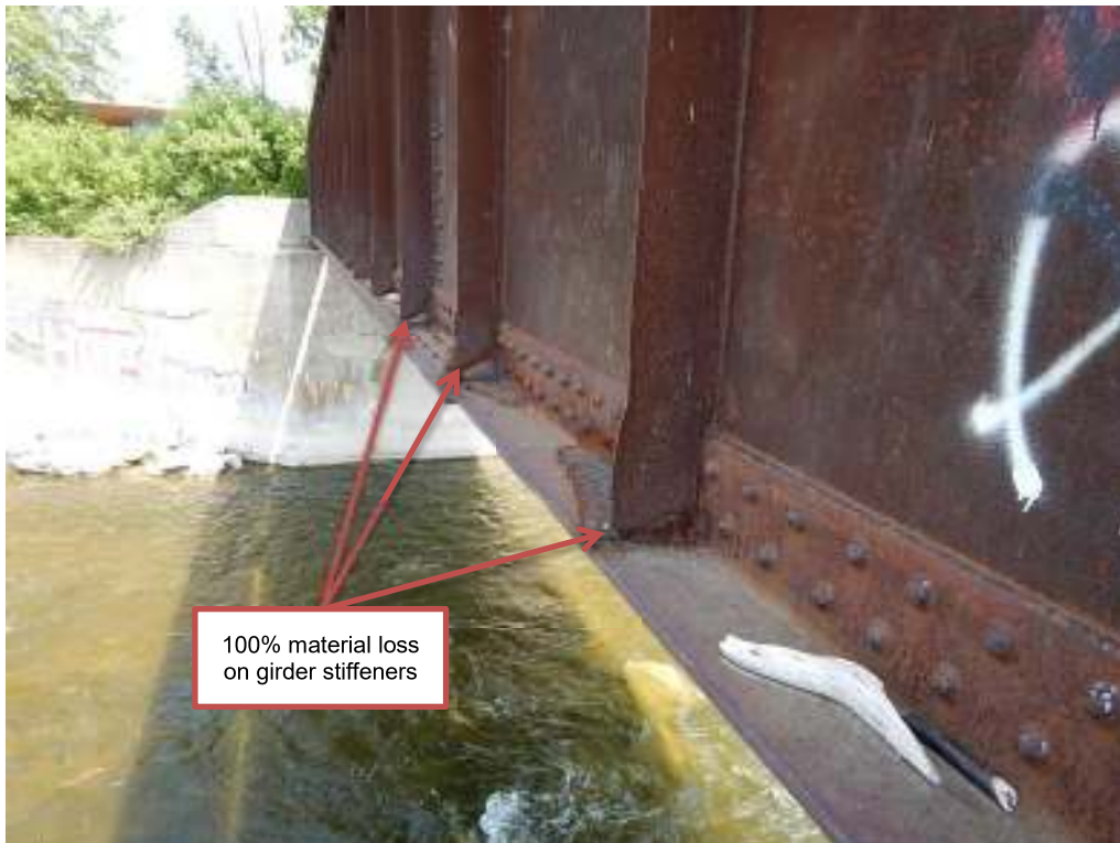
Photograph G10: East span, north girder exterior
