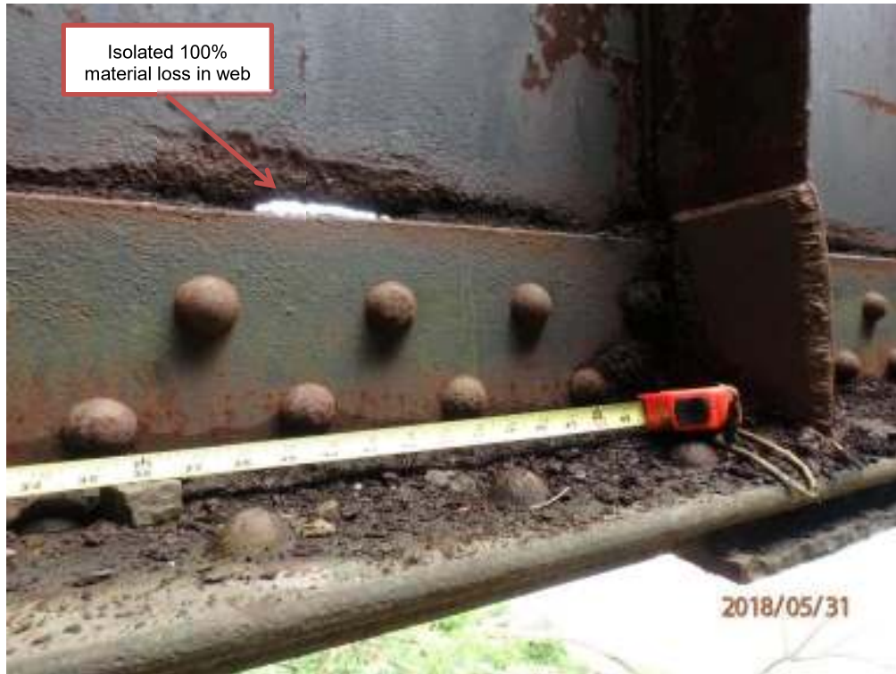
Photograph G7: West span, north girder
