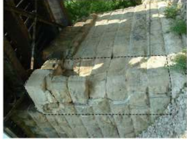
NORTH CORNER OF EAST ABUTMENT
