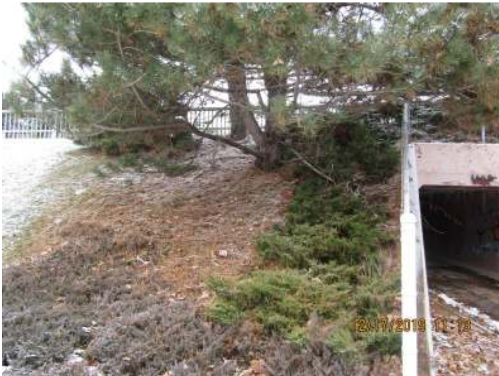
38 South west embankment
