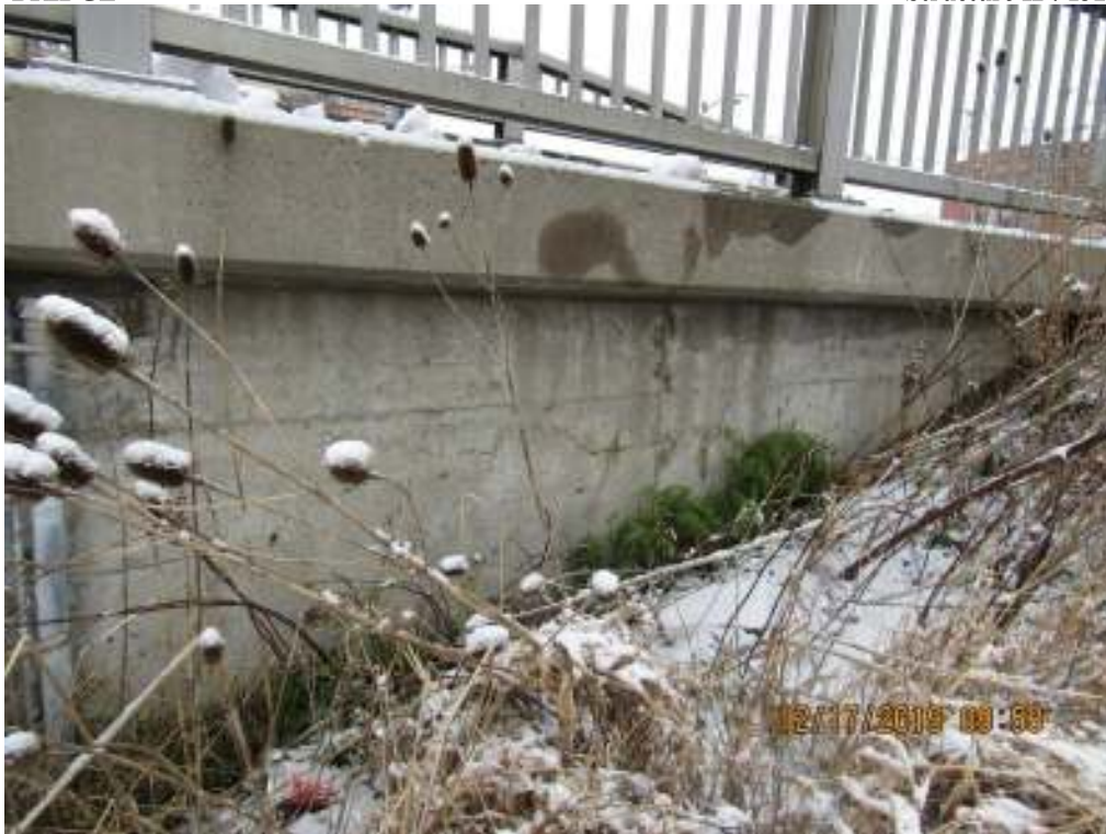
39 South east wingwall
