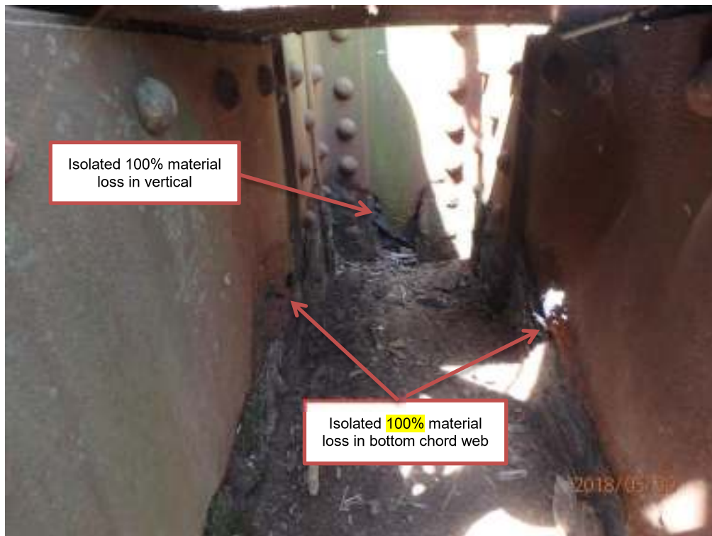
Photograph T8: Typical vertical connection at bottom chord
