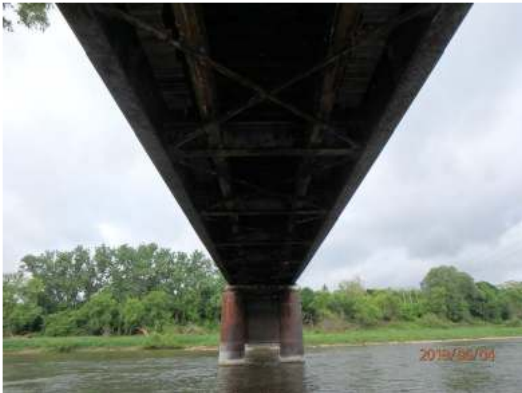
Photograph 14: Underside, looking west
