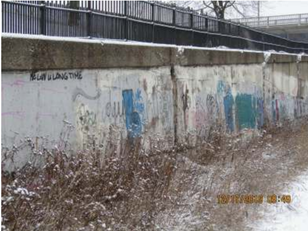
43 East retaining wall section north of bridge
