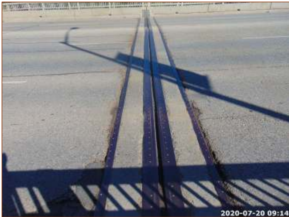
Photo 4 – West Expansion Joint
