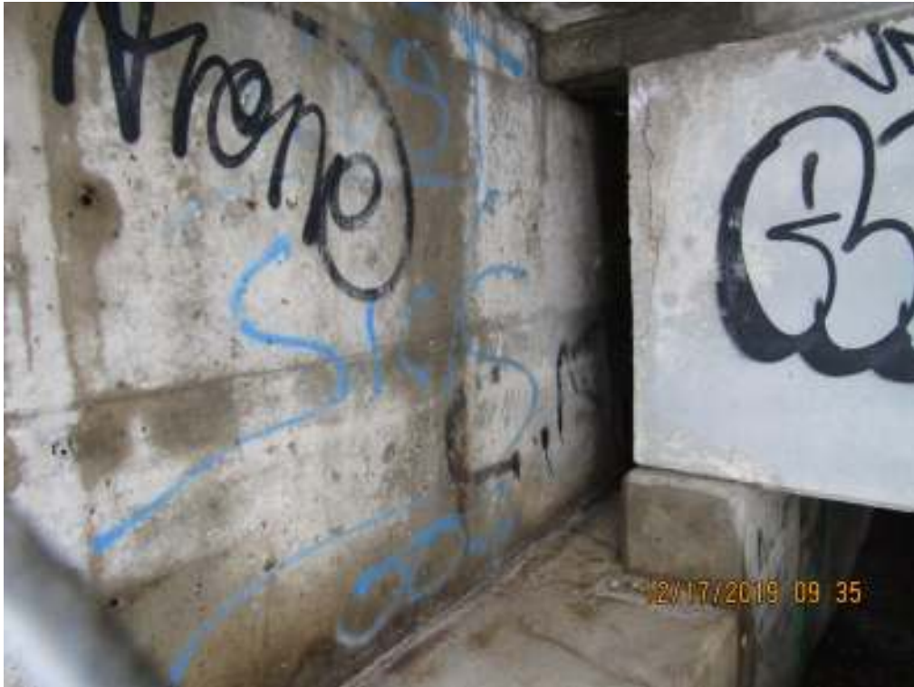
41 North ballast wall
