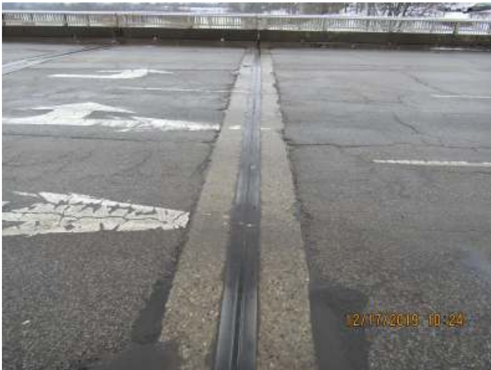
08 West expansion joint
