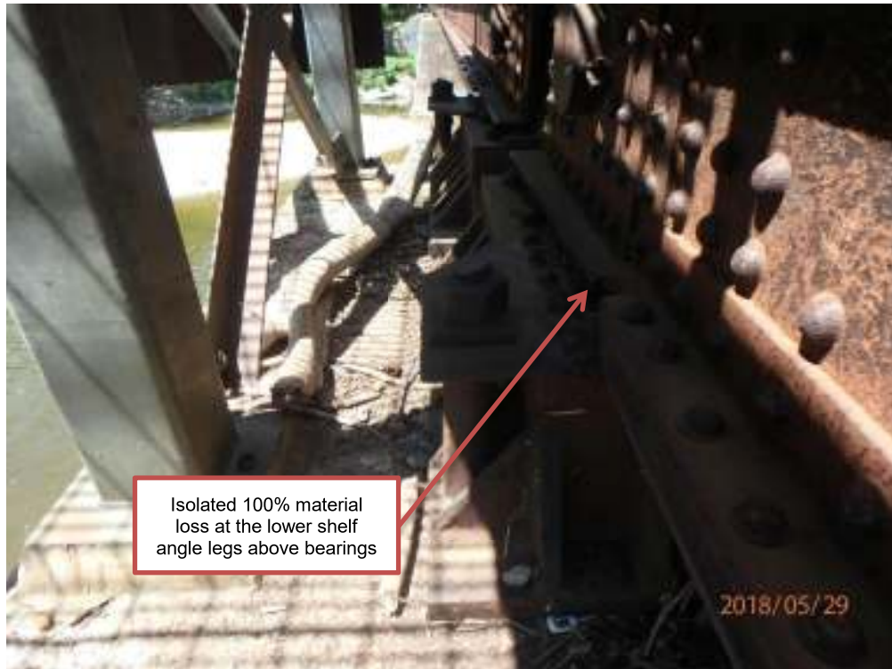
Photograph T6: Centre pier, southeast bearing
