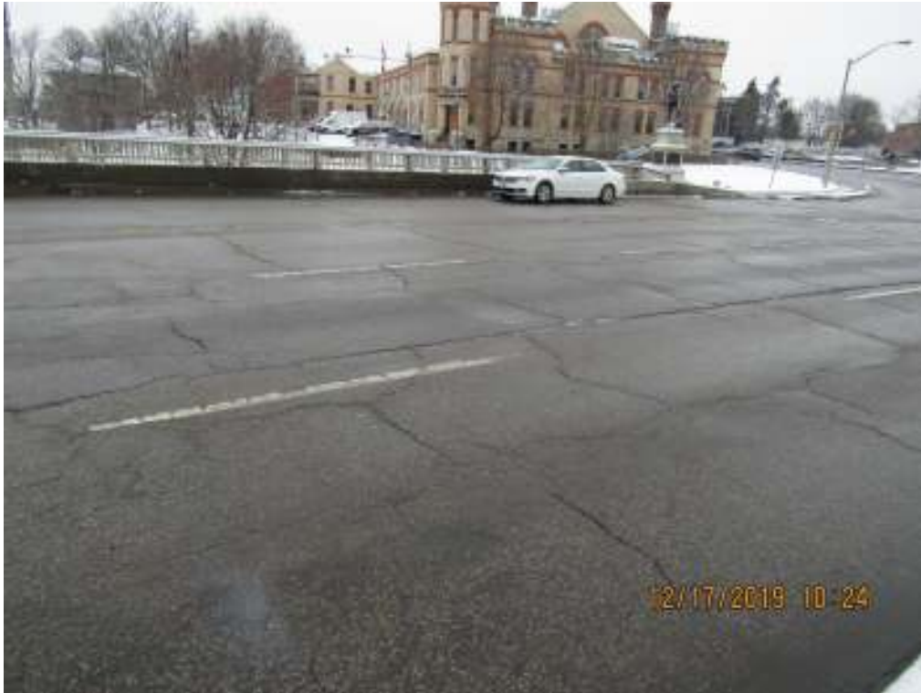
03 Deck, looking east
