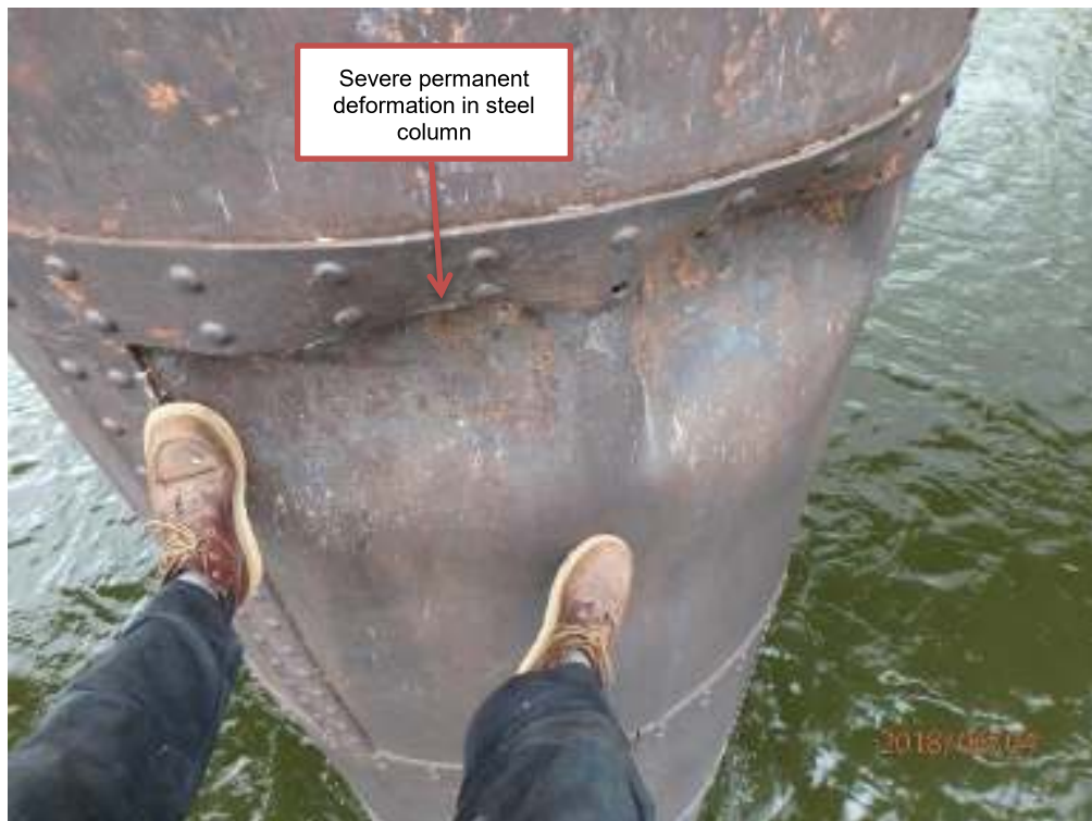
Photograph 8: Center pier, north steel column (north face)
