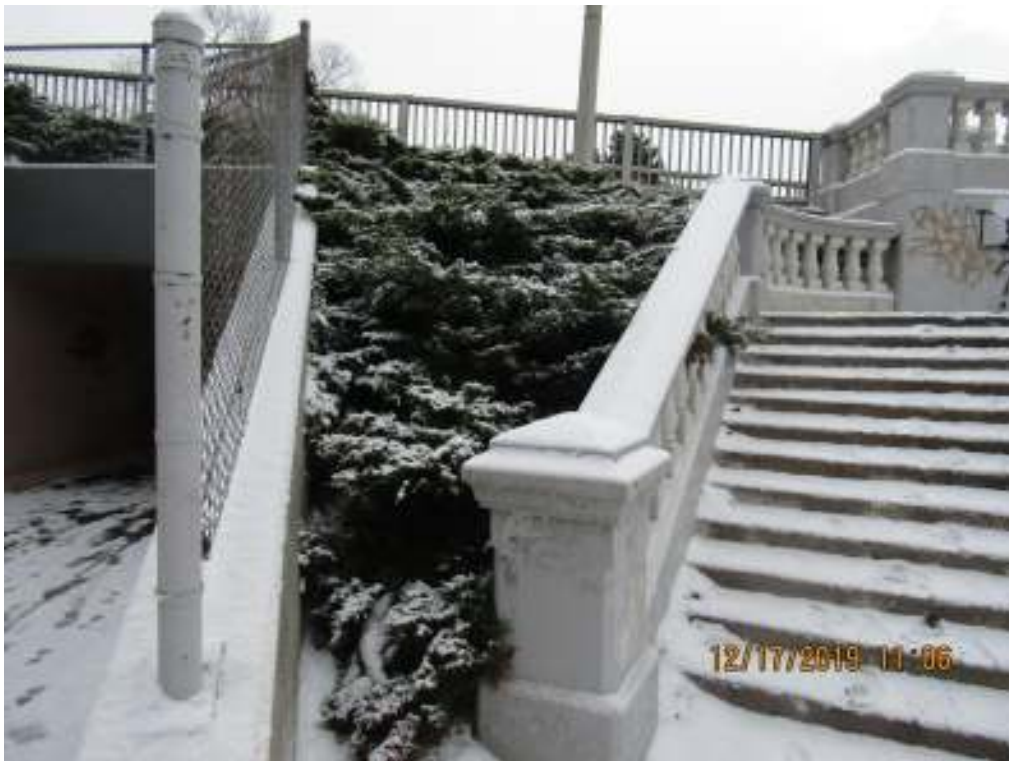
36 North west embankment
