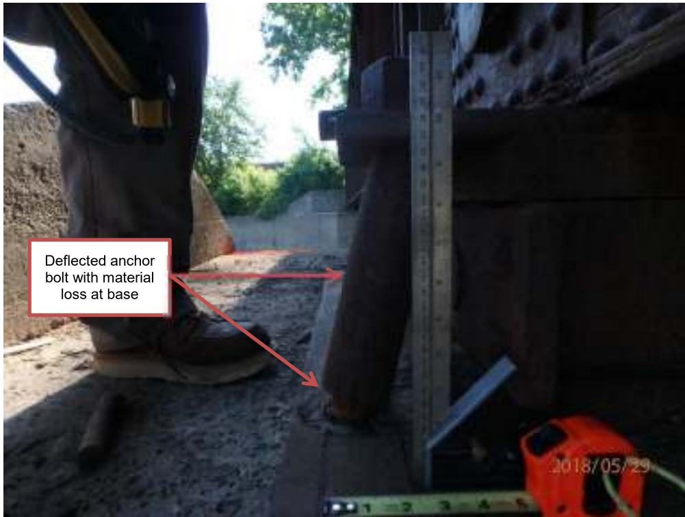
Photograph T3: East pier, north roller bearing
