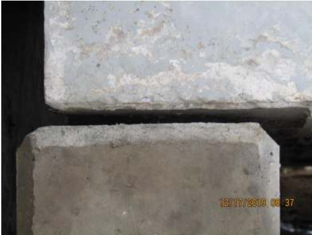
37 Typical north bearing
