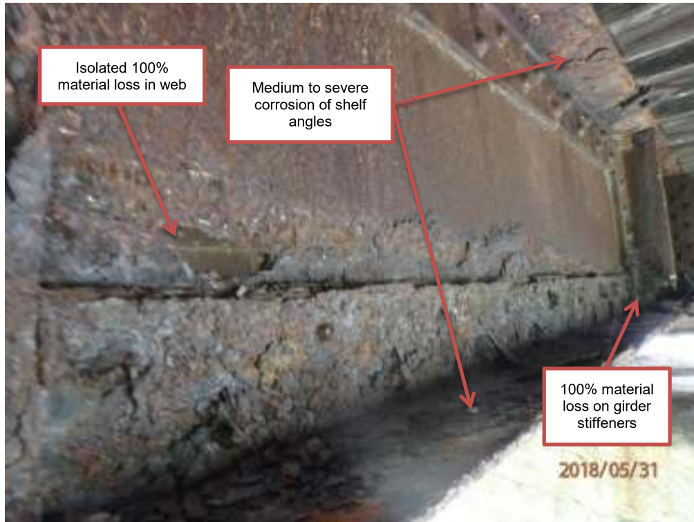
Photograph G11: West span, south stringer
