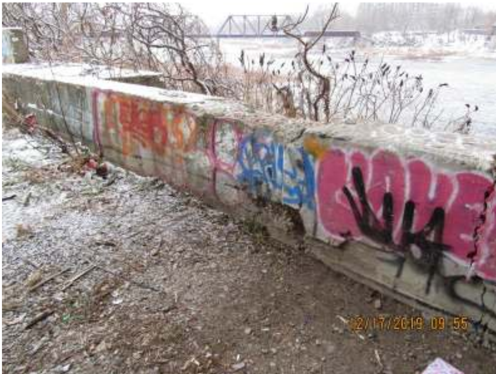
46 West retaining wall section south of bridge
