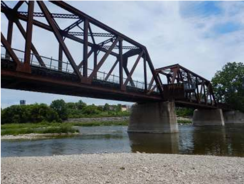
Photograph T1: Truss bridge span, south elevation
