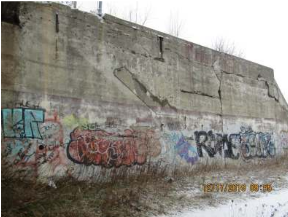
44 East retaining wall section south of bridge
