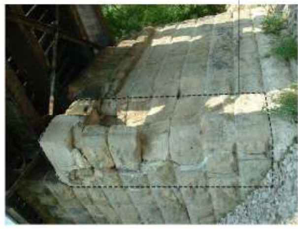
NORTH CORNER OF EAST ABUTMENT
