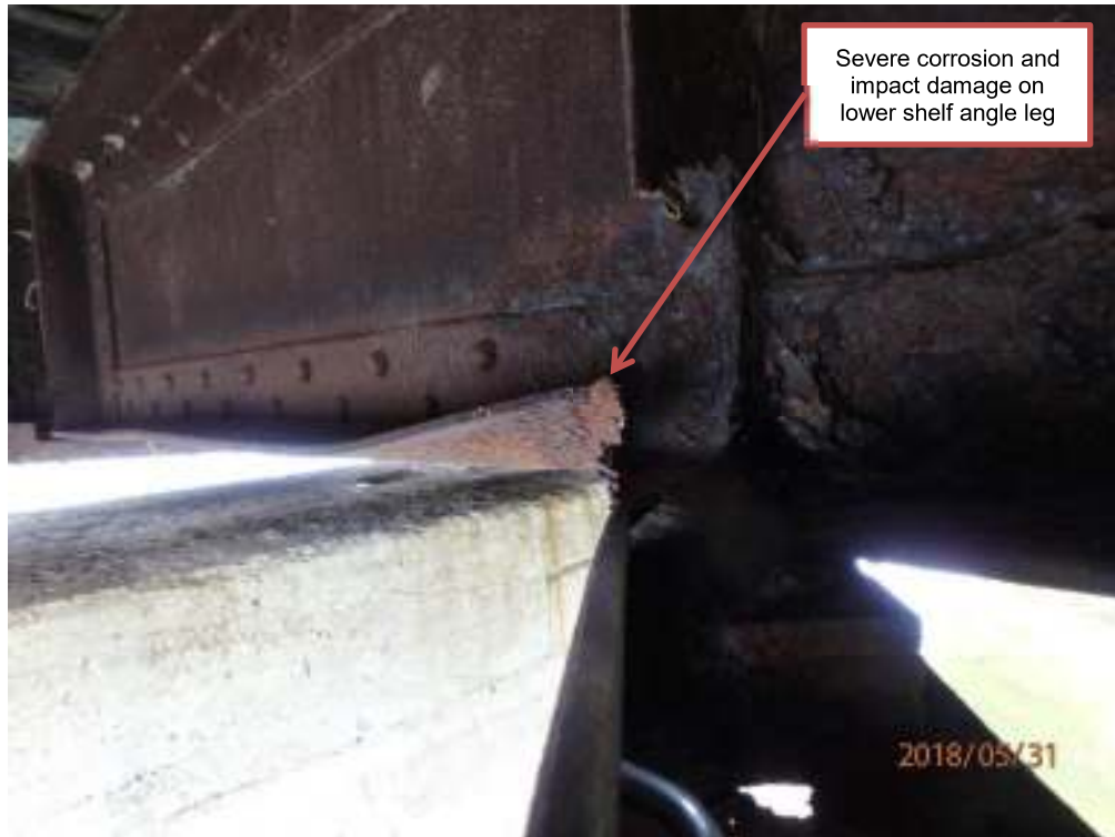
Photograph G12: West span, north stringer
