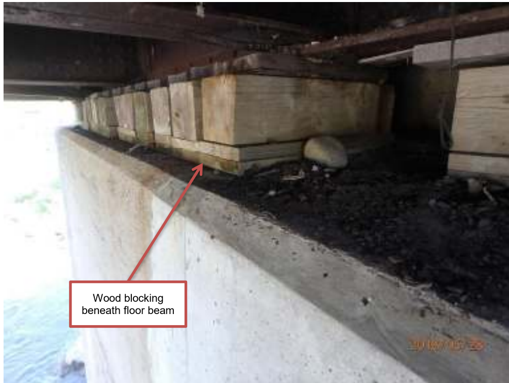
Photograph G3: East abutment
