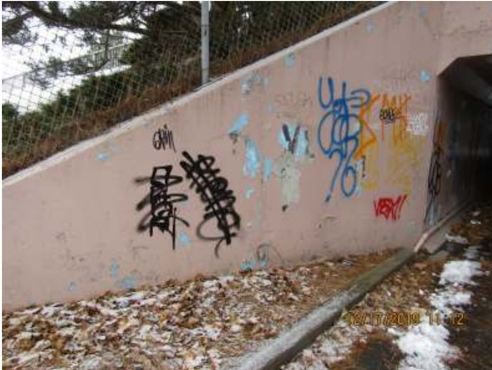
19 South west retaining wall
