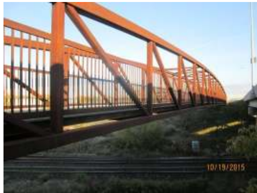
Figure 3: Prefabricated steel truss superstructure (Structure 152)
