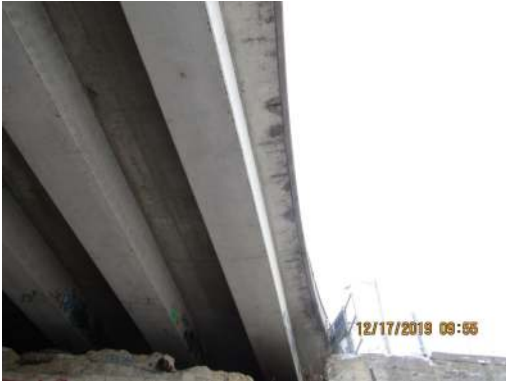
15 South exterior soffit
