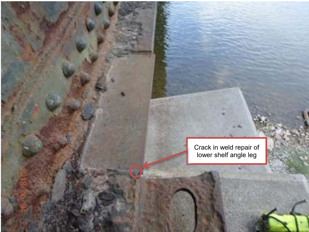
Photograph 16: North girder at east abutment
