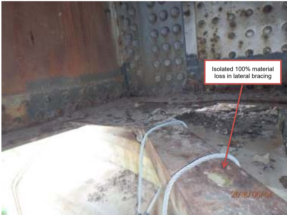
Photograph 18: East span, lateral bracing
