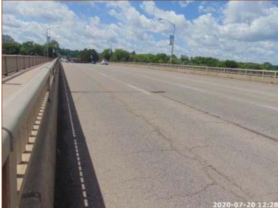
Photo 3 – Wearing surface, looking West
