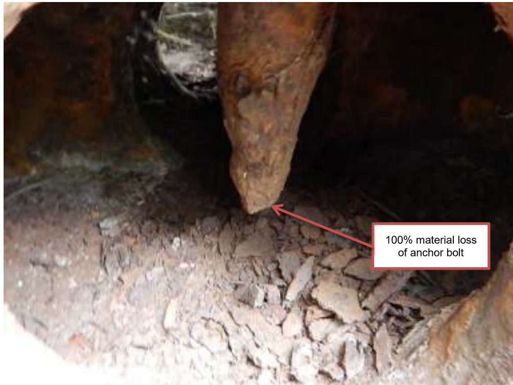
Photograph G6: West abutment, north bearing anchor bolt
