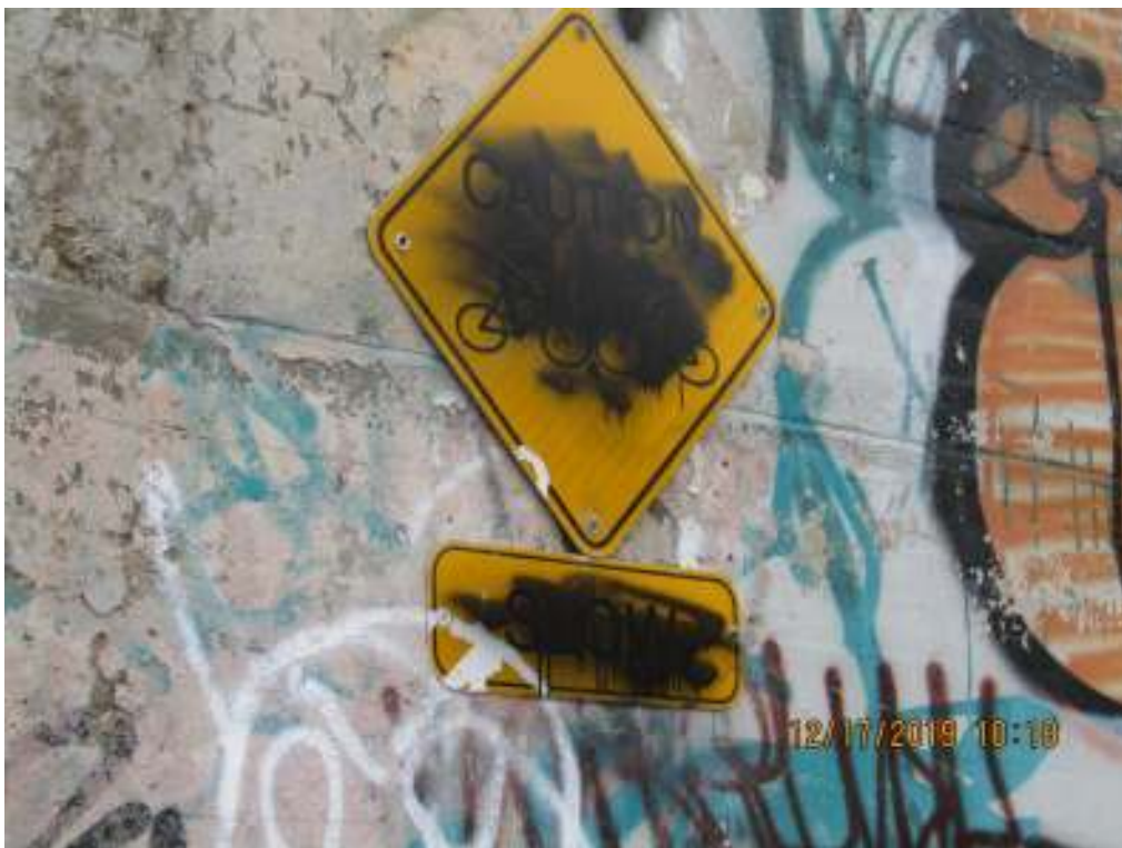
76 Sign on bridge
