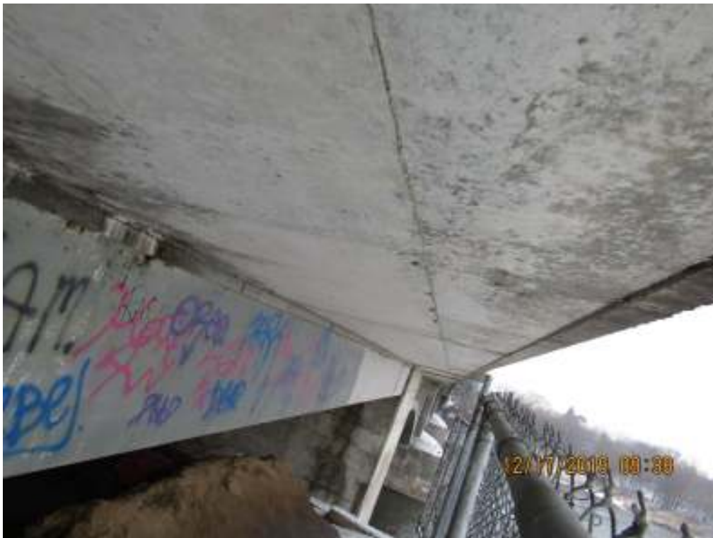
16 North exterior soffit
