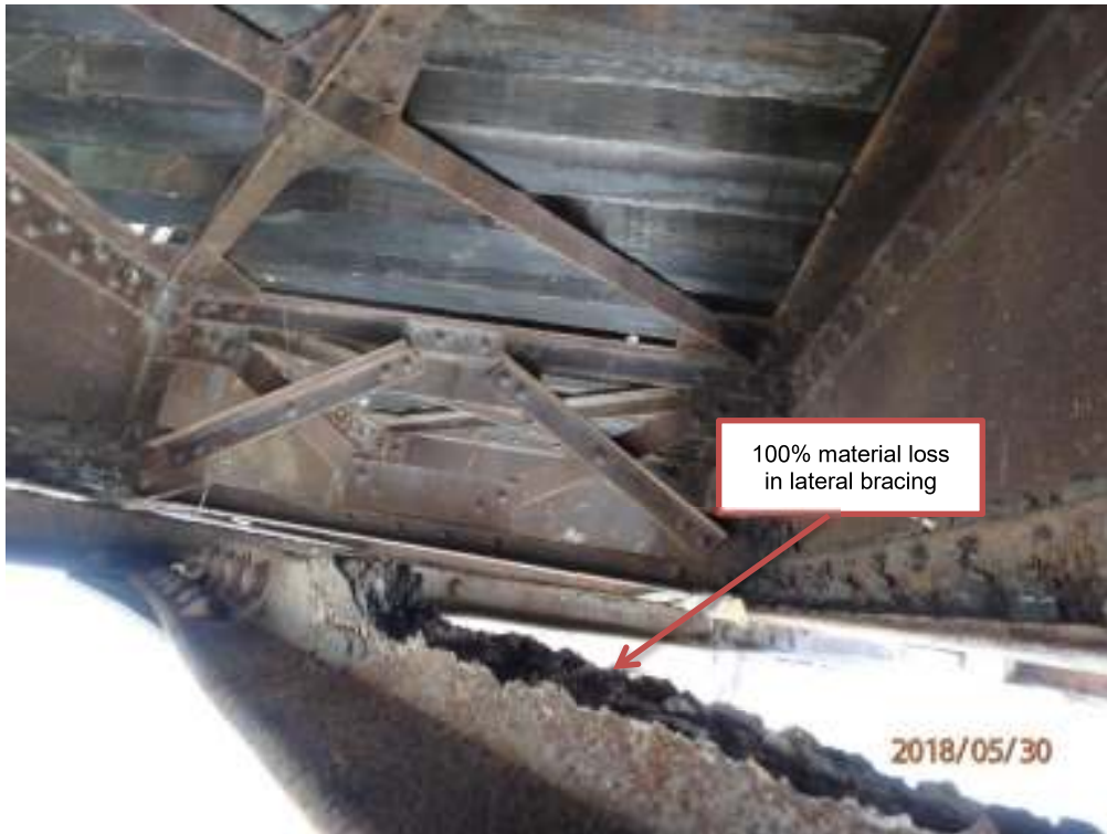
Photograph T13: East truss, lateral bracing
