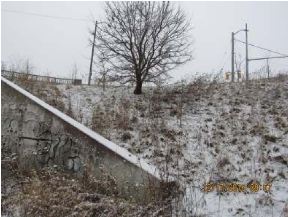
74 South east embankment
