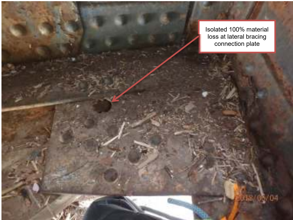
Photograph 17: East span, lateral bracing connection plate
