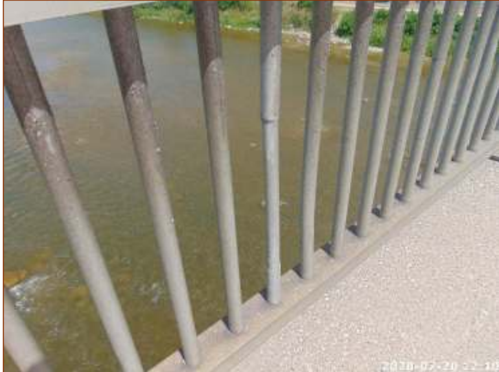
Photo 13 – North Exterior Railing, Typical Spindle Repair
