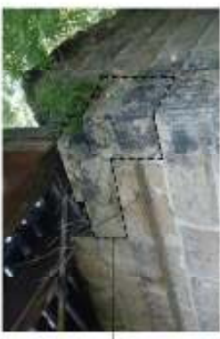
SOUTH CORNER OF EAST ABUTMENT
