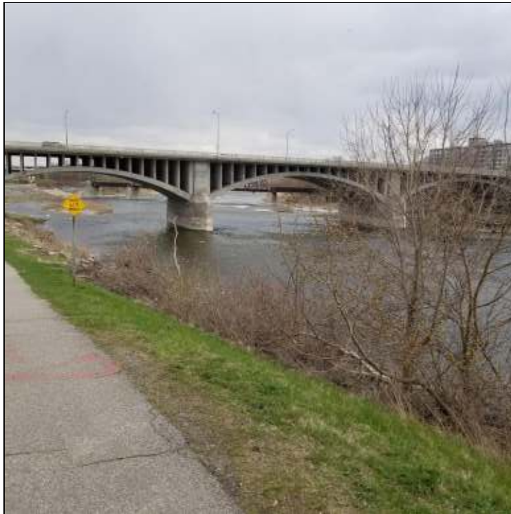
Photograph 1: View of Lorne Bridge, looking south.
