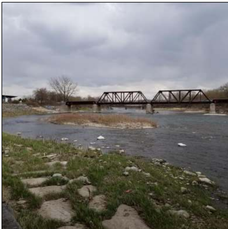
Photograph 4: View along the east bank of the river, looking south. Brant's Crossing Bridge in the background.
