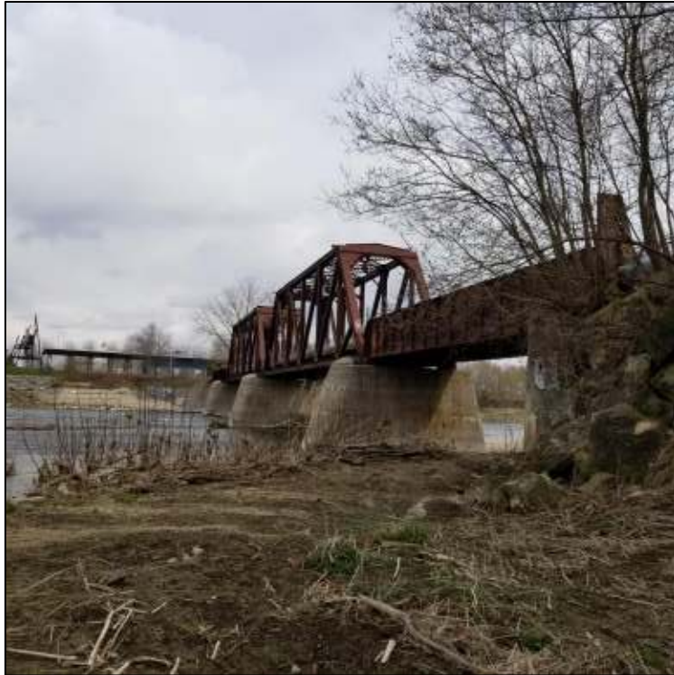
Photograph 3: View of the Brant Crossing Bridge, looking east.
