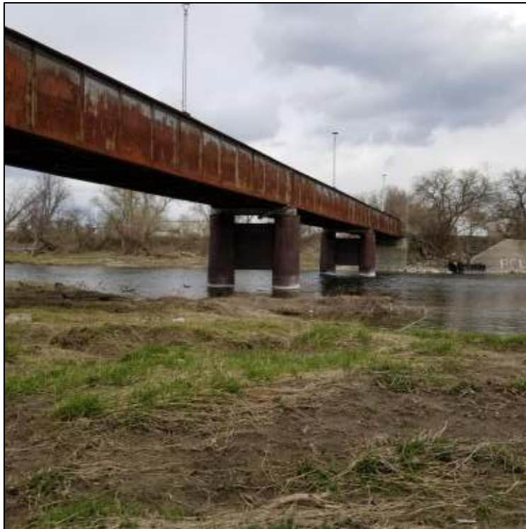
Photograph 5: View of the TH&B Railway River Crossing, looking east.
