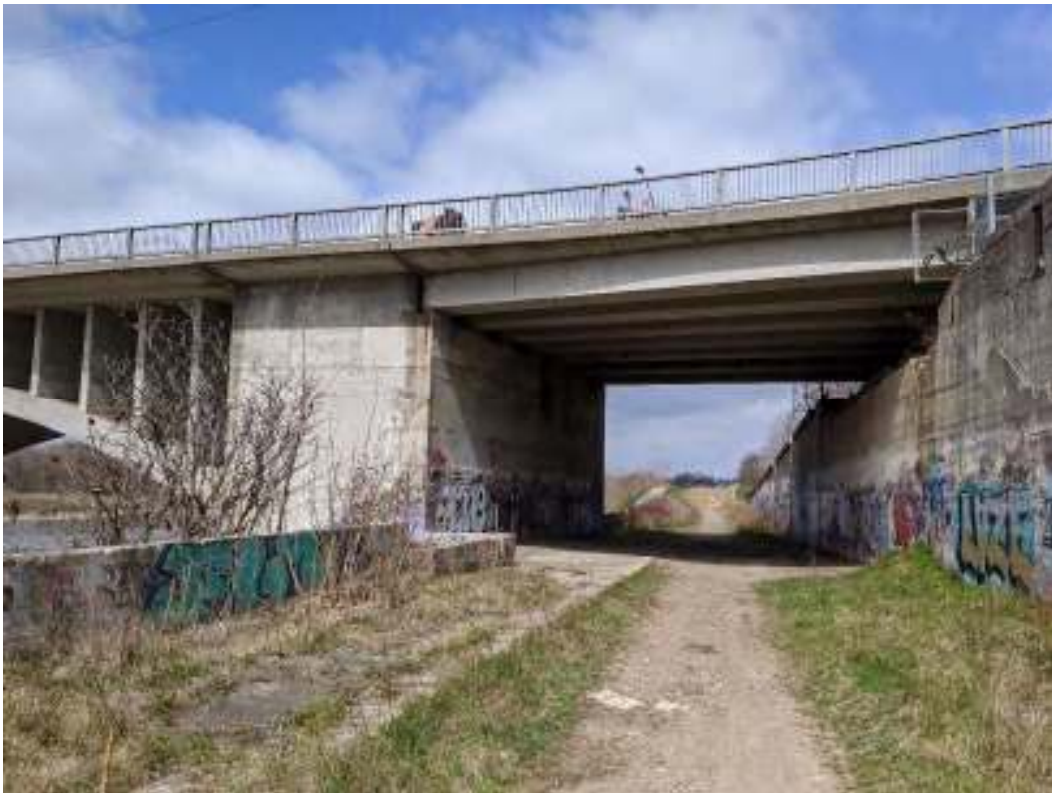
Figure 41: The Lorne Bridge Girder Span that forms the east approach of the Lorne Bridge
