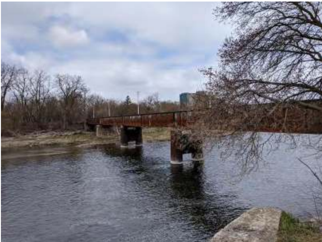
Figure 134: View facing northwest of the girder spans
