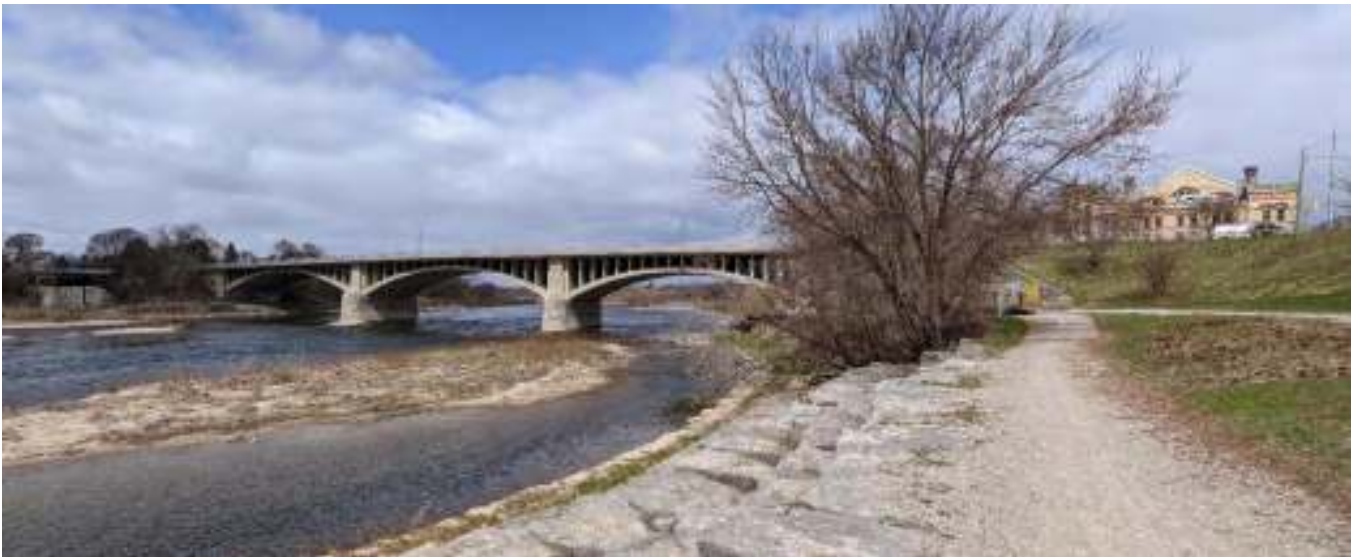
Figure 31: View of the Lorne Bridge facing north from the east bank
