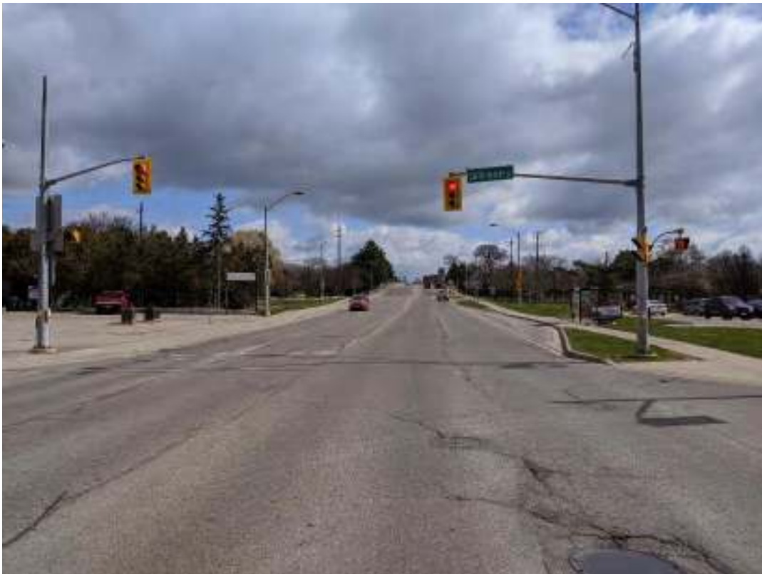
Figure 35: View facing east of the west approach
