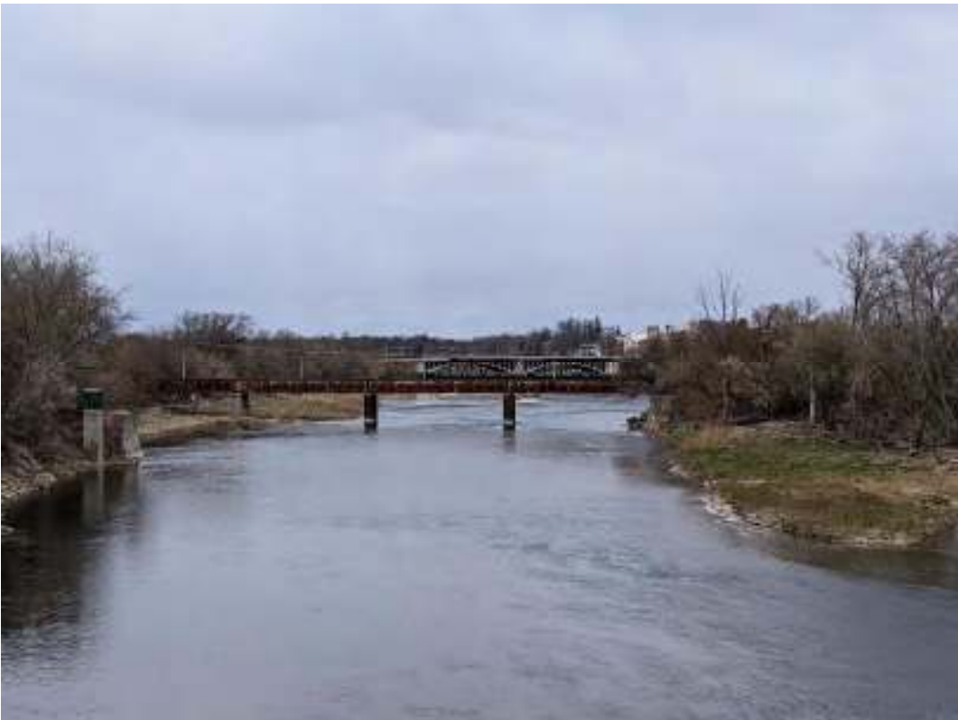
Figure 117: Setting of the TH&B Crossing Bridge, facing north from the BSAR Bridge
