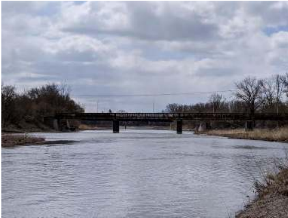
Figure 85: View downriver of the TH&B Crossing Bridge
