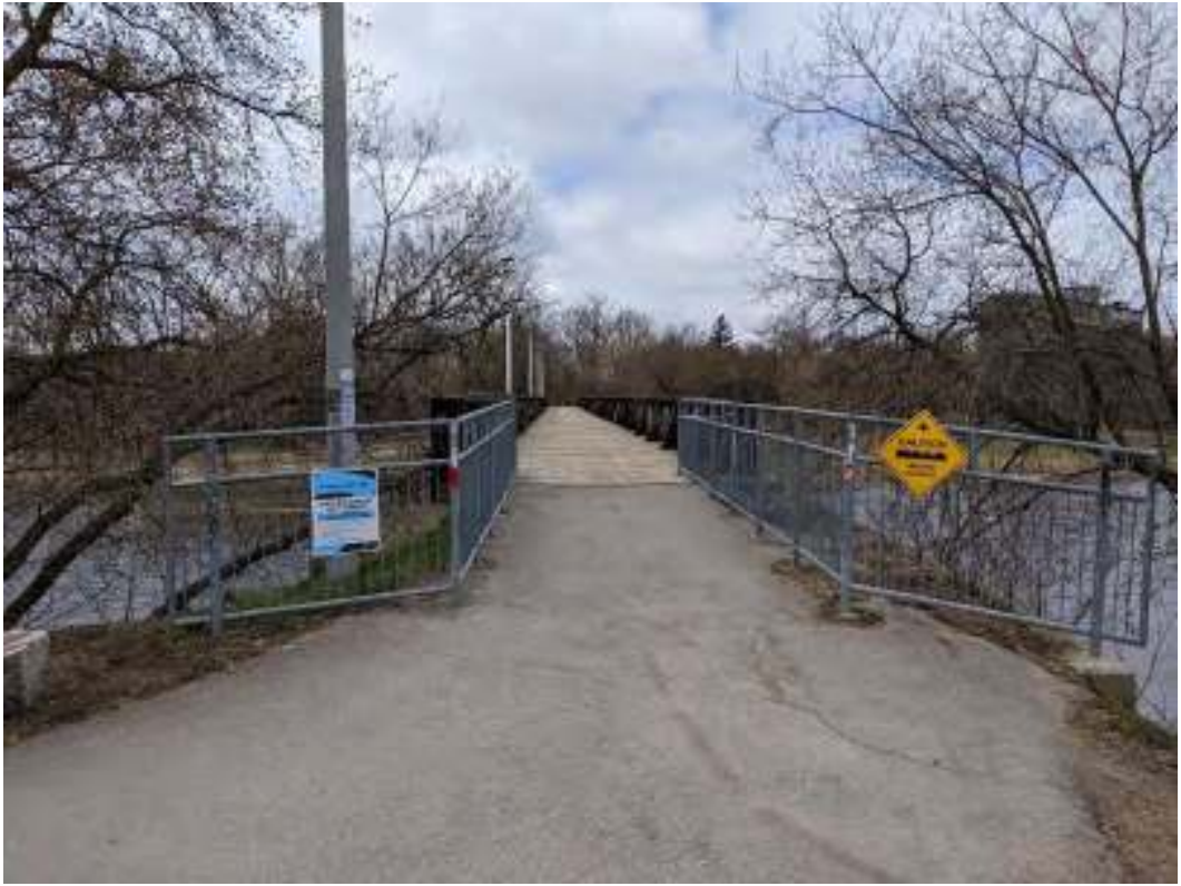
Figure 118: East approach to the TH&B Crossing Bridge, facing west
