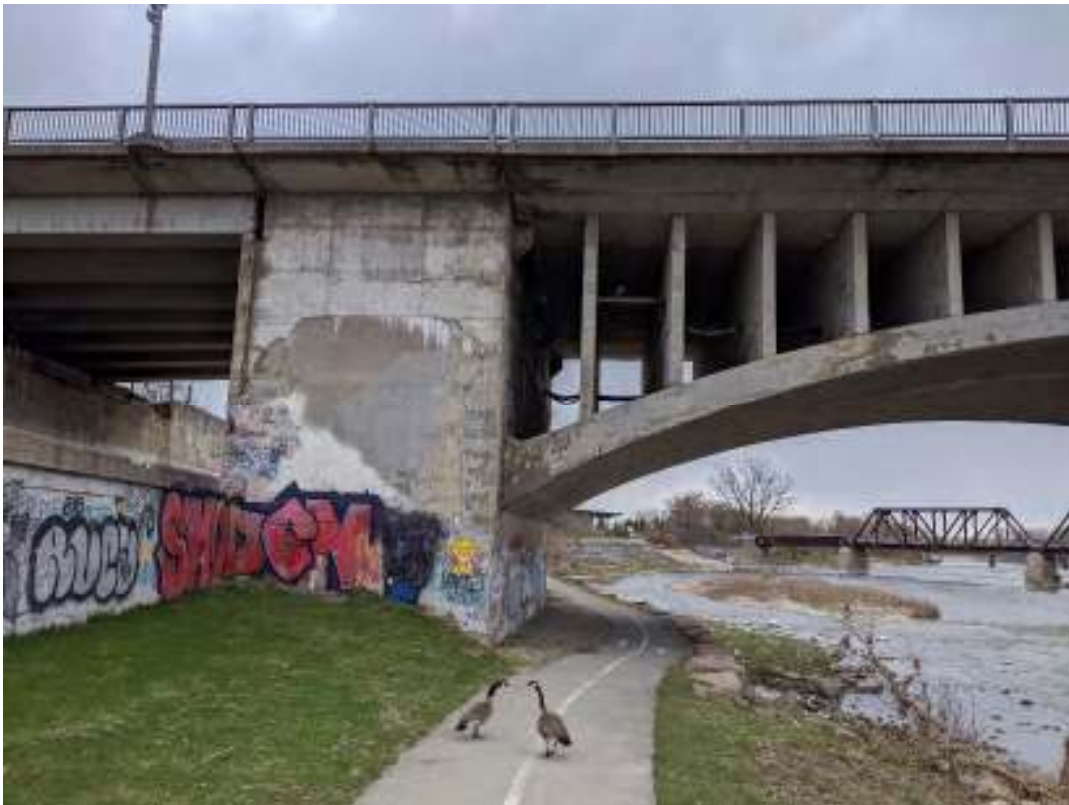
Figure 43: North side of the east abutment of the Lorne Bridge
