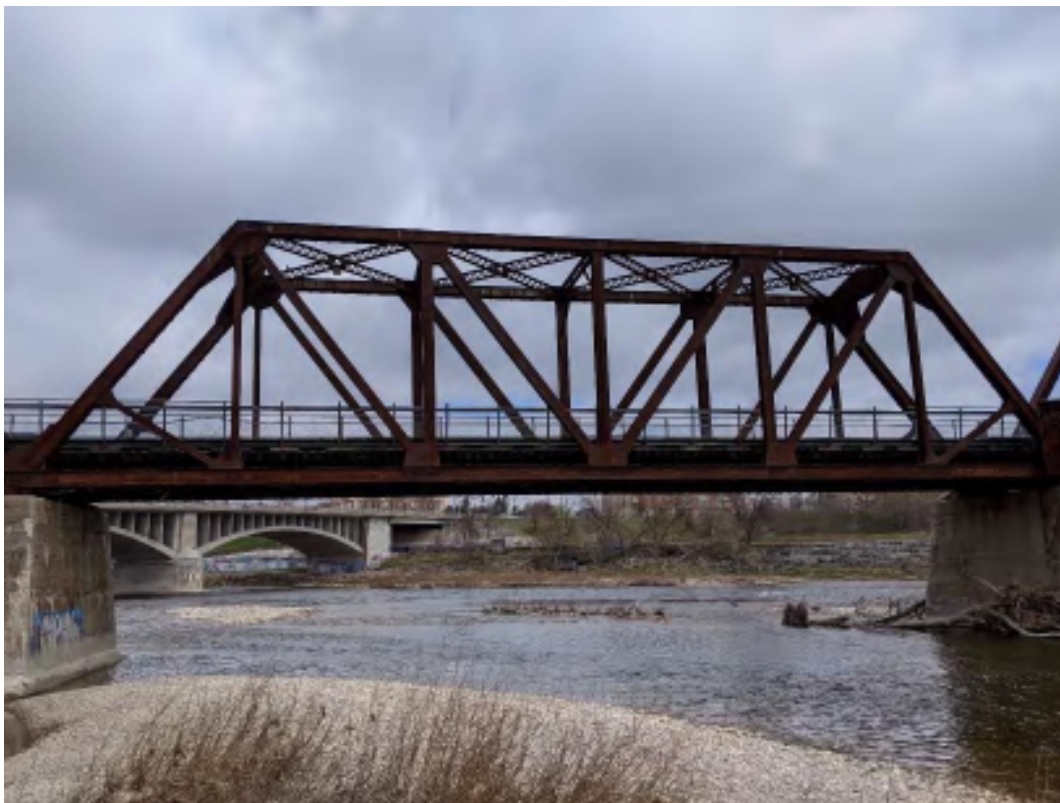
Figure 97: South side of the west Pratt through truss span
