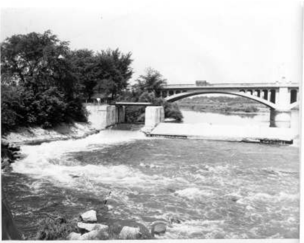
Figure 16: View facing north of the dam spillway, June 1954 (City of Brantford)
