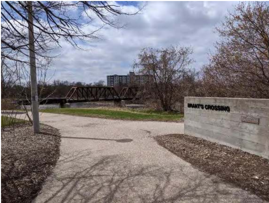
Figure 83: View from the Brant's Crossing entrance off Icomm Drive, facing southwest.
