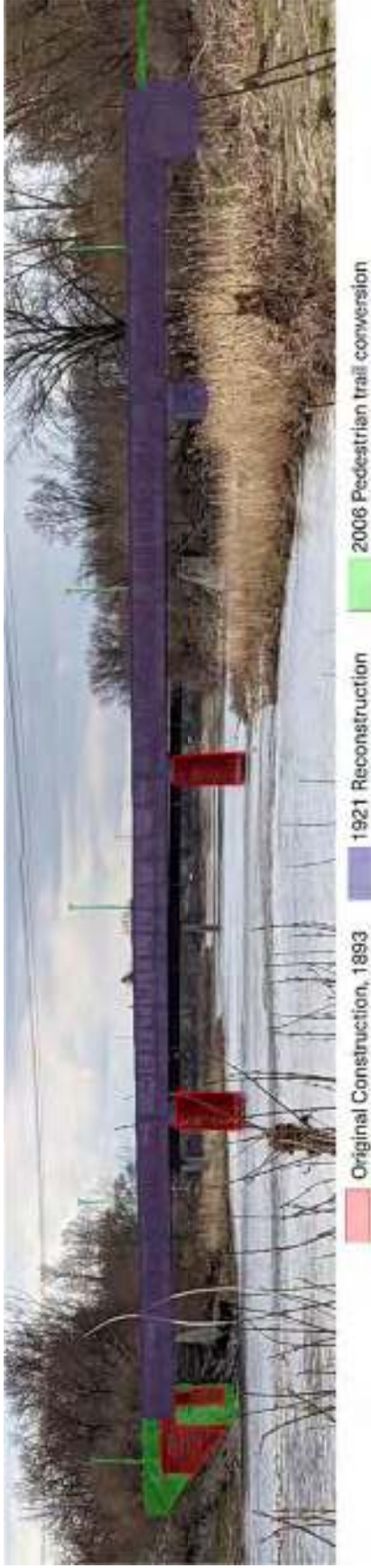
Figure 145: Visual integrity analysis of the TH&B Crossing Bridge
