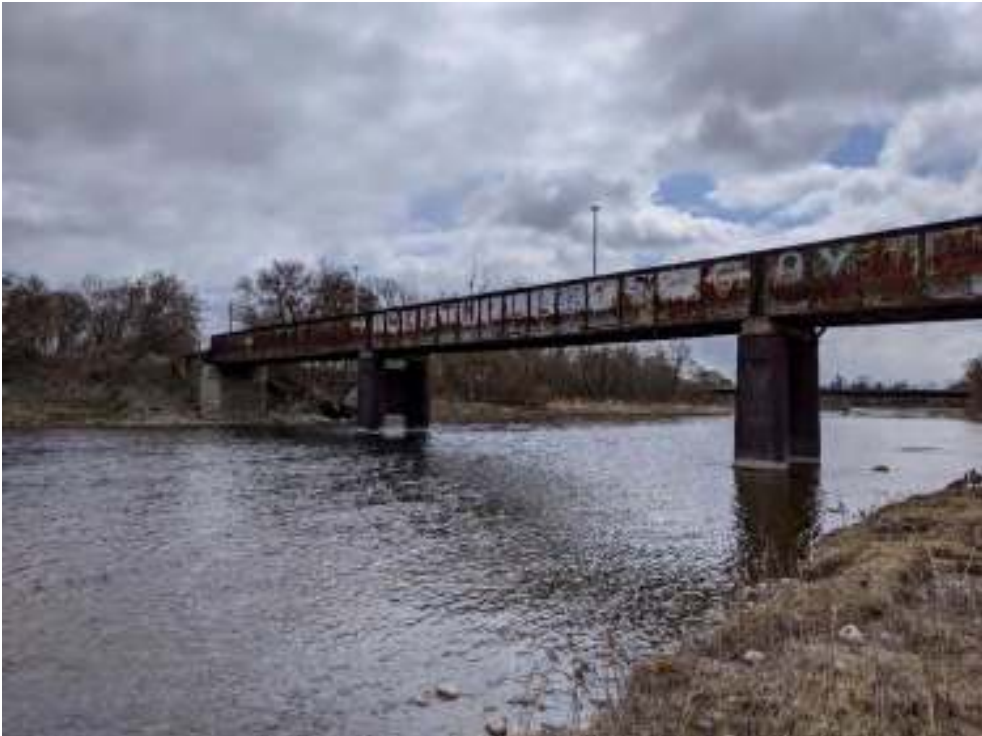
Figure 130: View facing southeast of the metal pier bents
