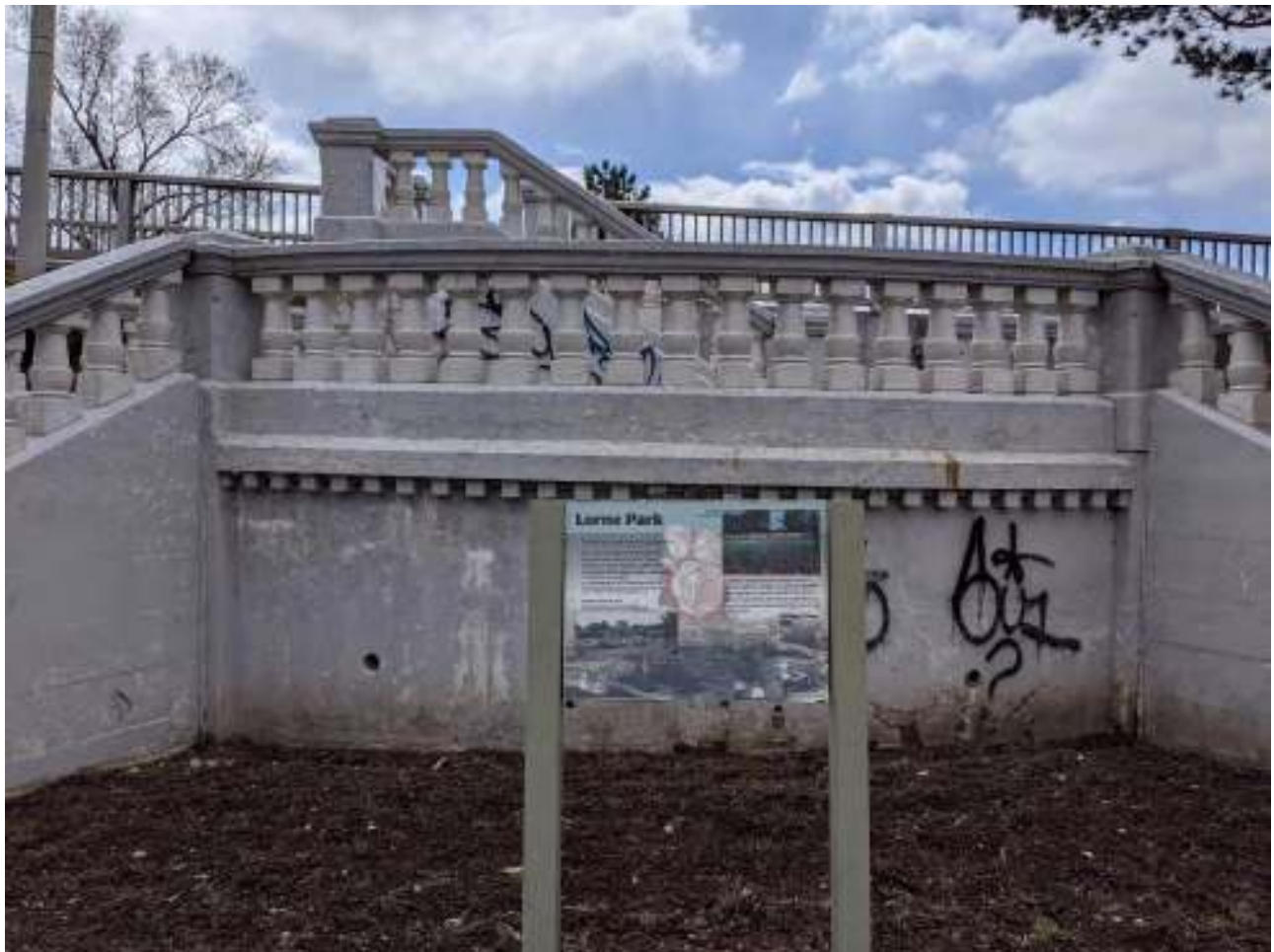
Figure 53: Outer face of the landing with denticulated cornice, thick square newels, and low chamfered and moulded handrail with “Renaissance” balusters
