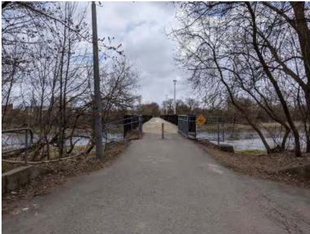
Figure 119: West approach to the TH&B Crossing Bridge, facing east
