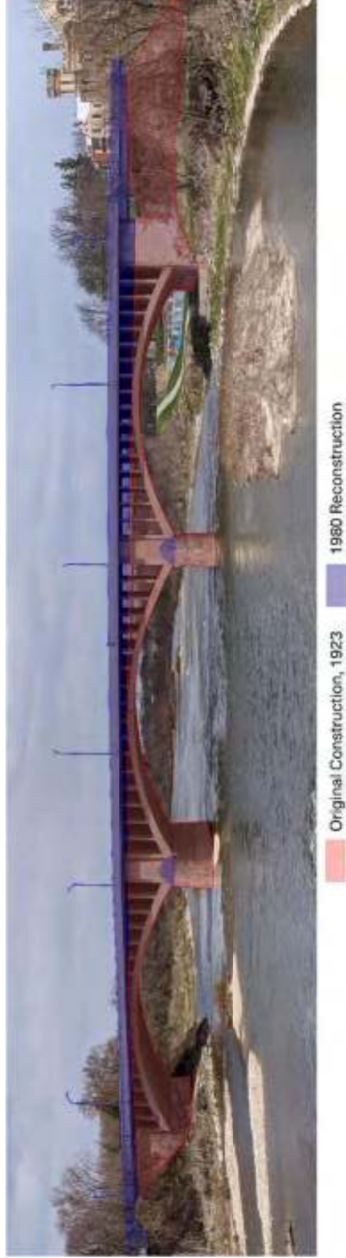
Figure 77: Visual integrity analysis of the Lorne Bridge
