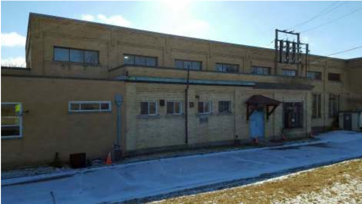
Figure 63: Pump Room at the Brantford Water Works, designed by Adams in 1931 (Golder 2016)
