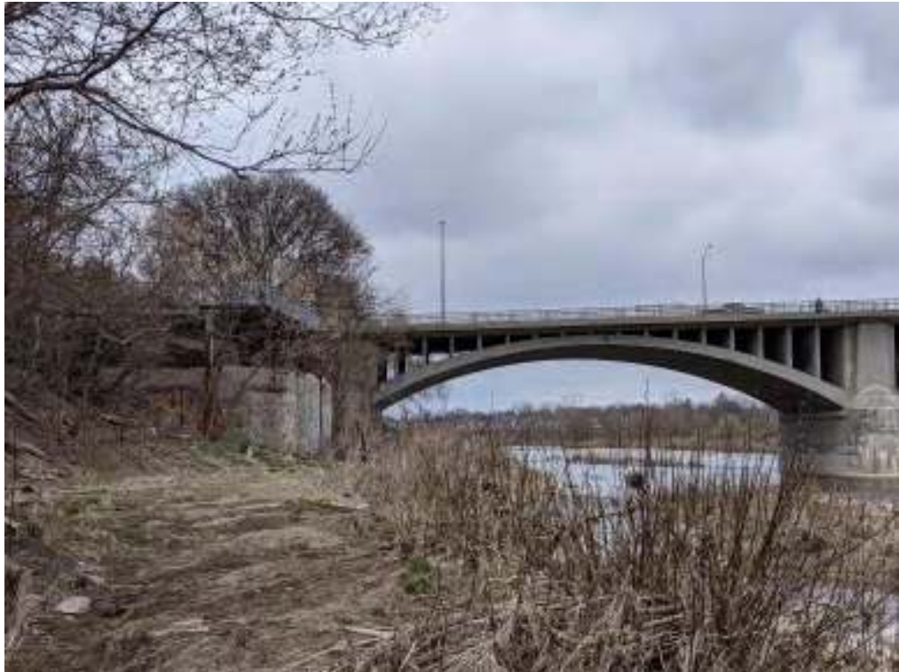
Figure 17: View facing north of the same area shown in Figure 16
