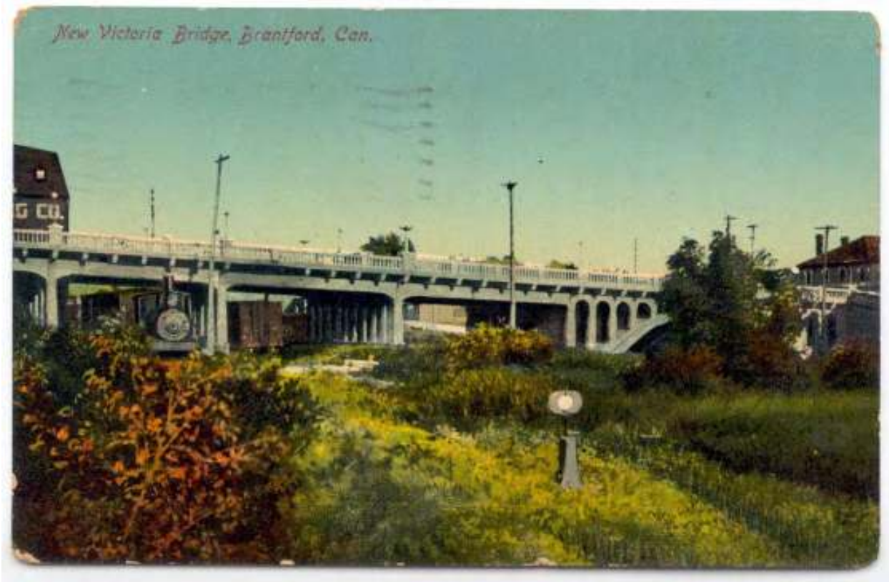
Figure 65: The 1912 New Victoria Bridge (Brantford Public Library)
