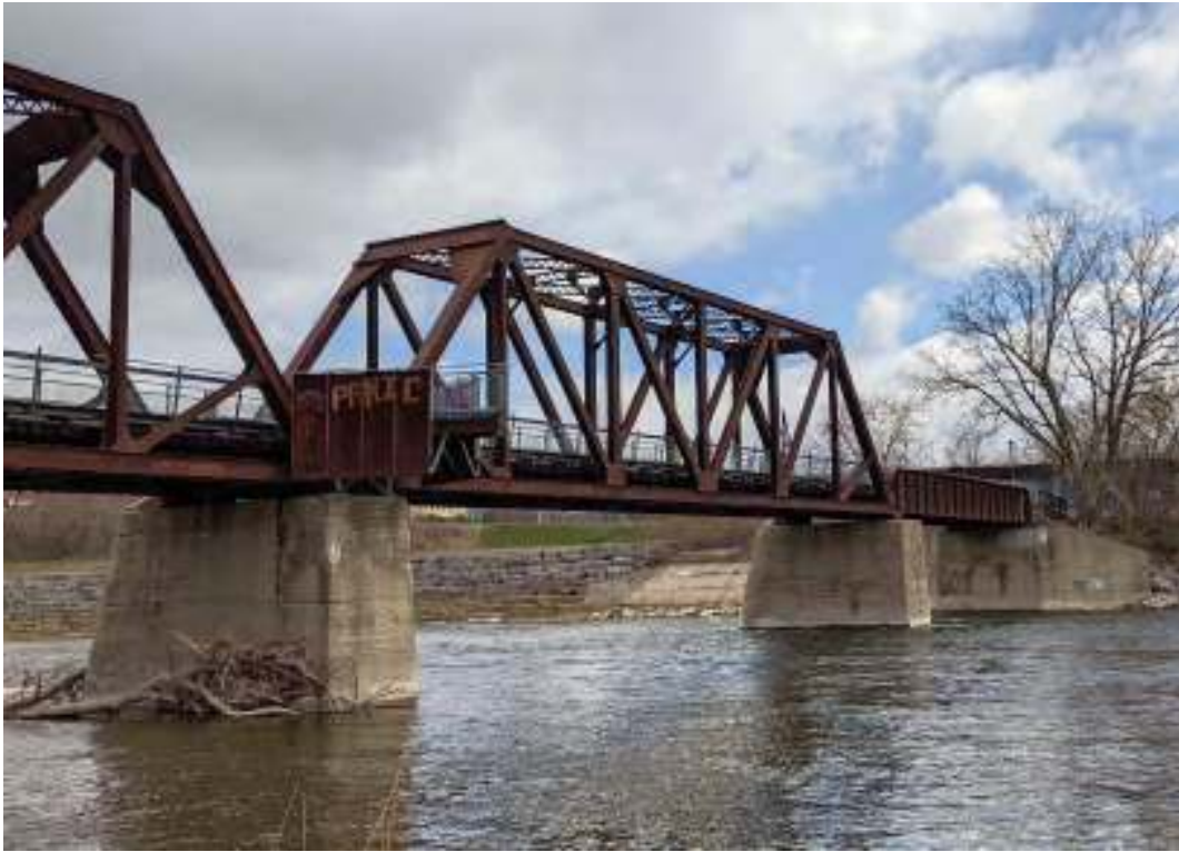
Figure 98: West and south sides of the east Pratt through truss span
