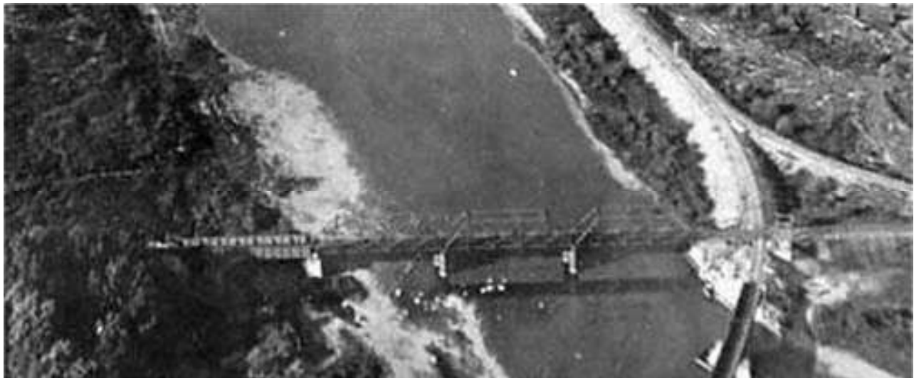
Figure 142: Detail from a 1919 oblique aerial photograph of the TH&B Crossing Bridge (Collection of Brant Railway Heritage Society)
