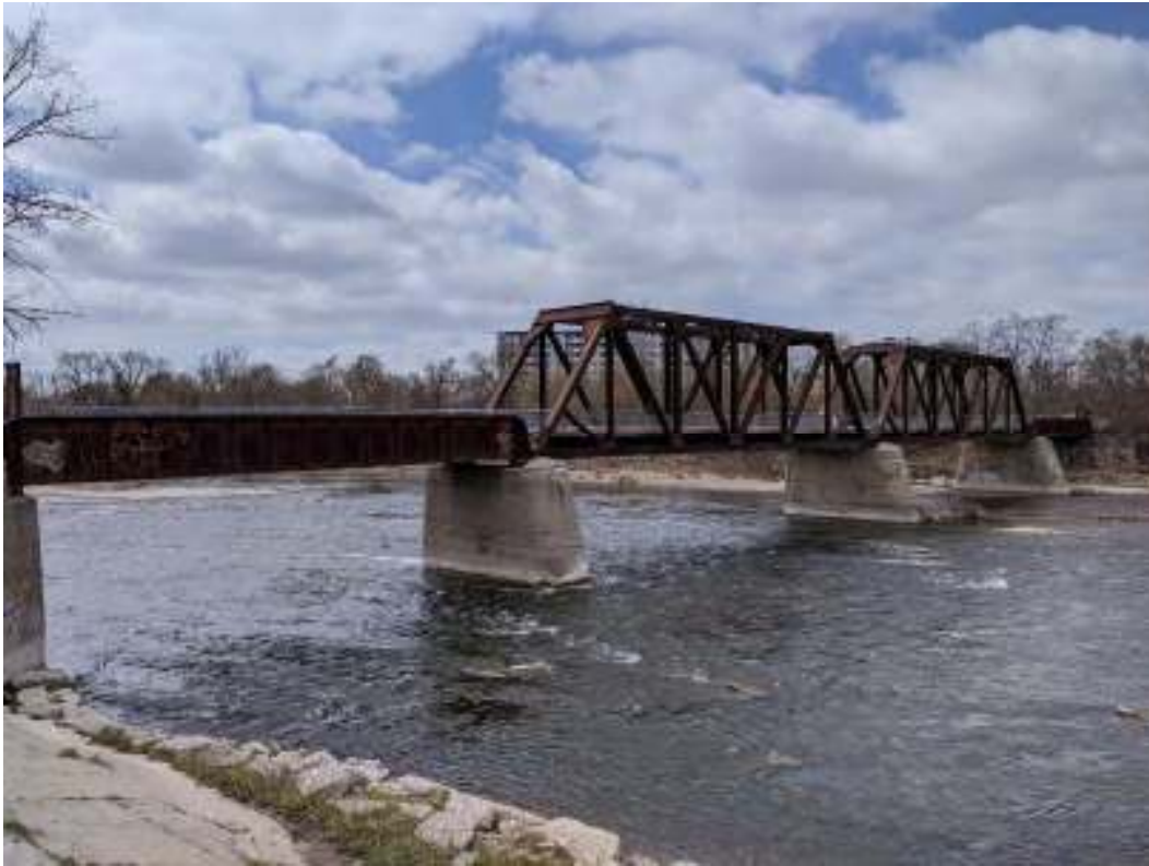
Figure 89: Upriver side of the piers, facing southwest
