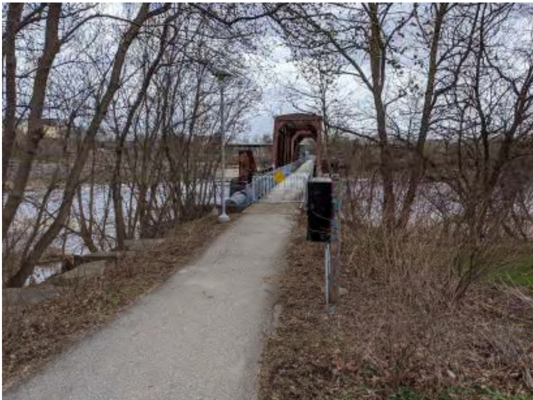
Figure 82: West approach to Brant's Crossing
