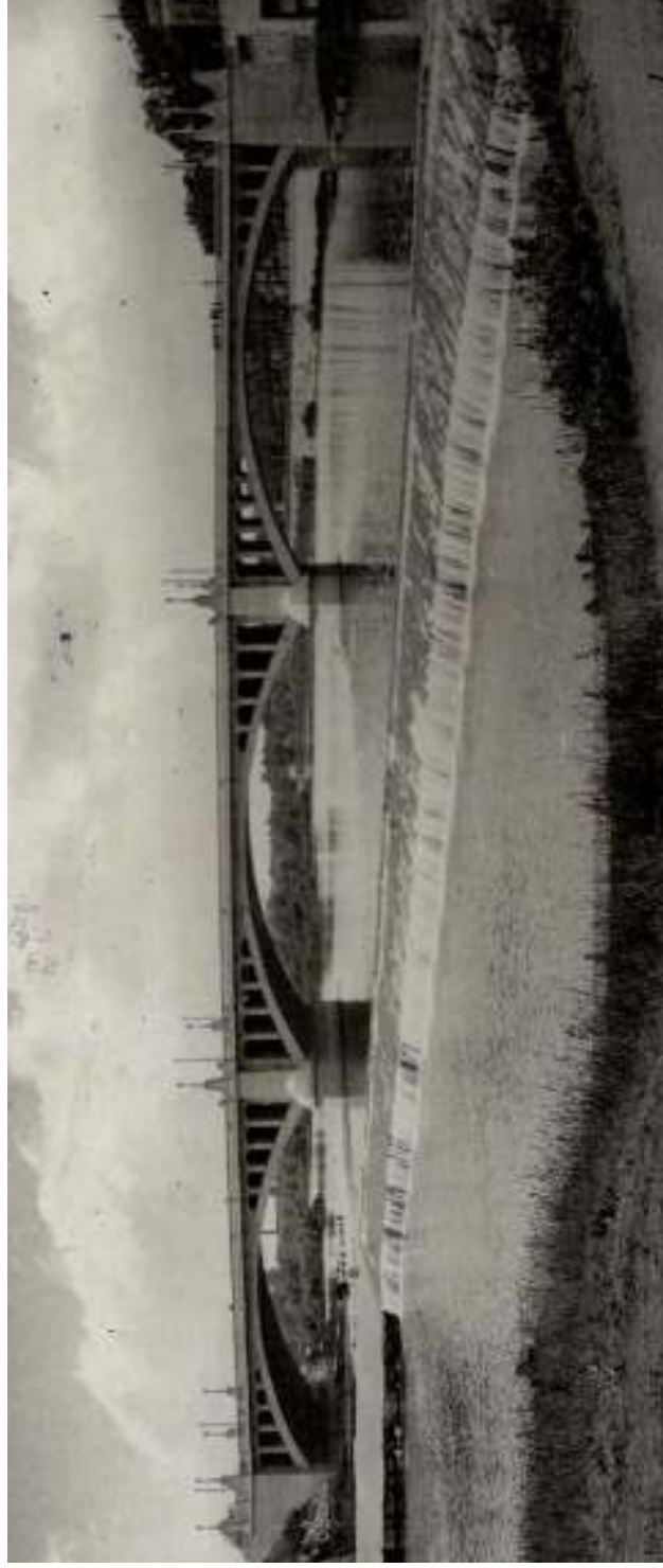
Figure 67: The Old Southwark Bridge spanning the Thames in London England, built in 1819 and replaced in 1921 (Historic England). Note the shallow arch spans, mouldings at the top of the sharp-nosed piers, and prominent parapet posts over the piers that match those of the Lorne Bridge (see Figure 68)
