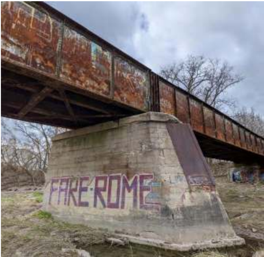
Figure 129: View facing south of the concrete pier
