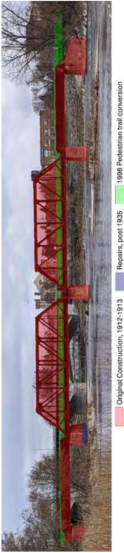
Figure 115: Visual integrity analysis of Brant's Crossing Bridge
