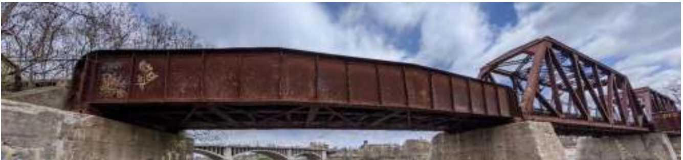
Figure 92: West approach girder span (includes some camera distortion).
