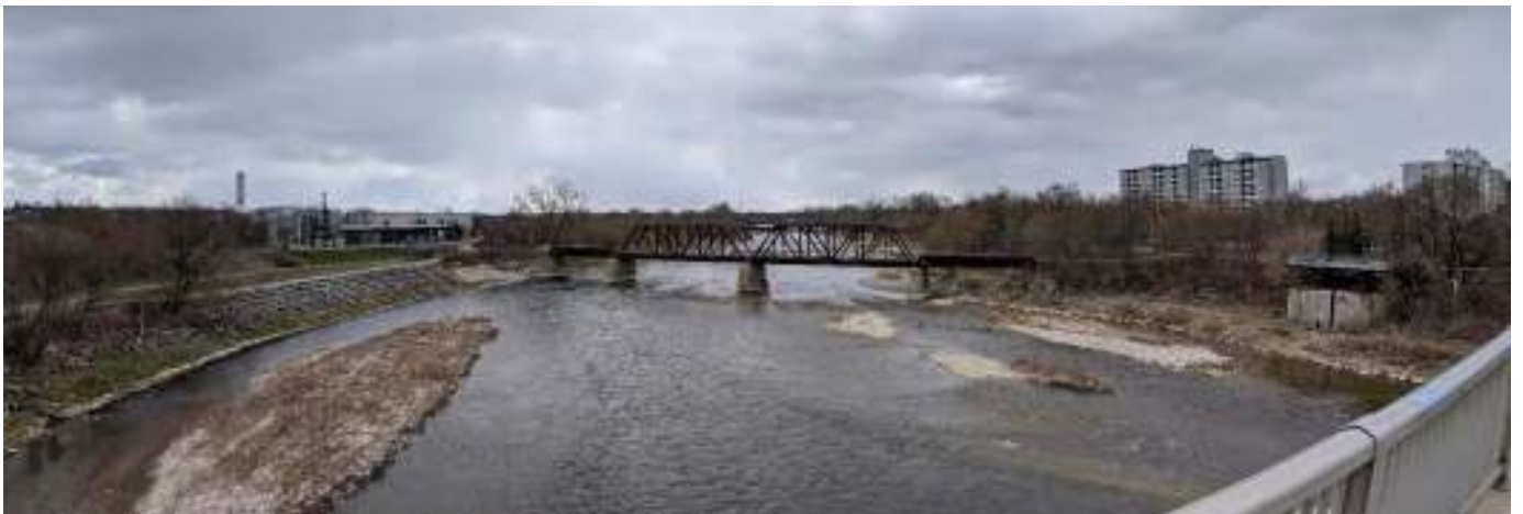
Figure 38: Vista facing south from the Lorne Bridge
