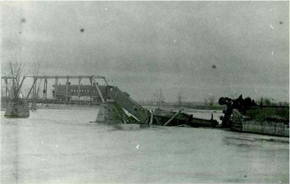
Figure 106: Bridge collapse and BN&PB Railway train derailment at the Brant's Crossing site, November 9, 1877 (courtesy)
