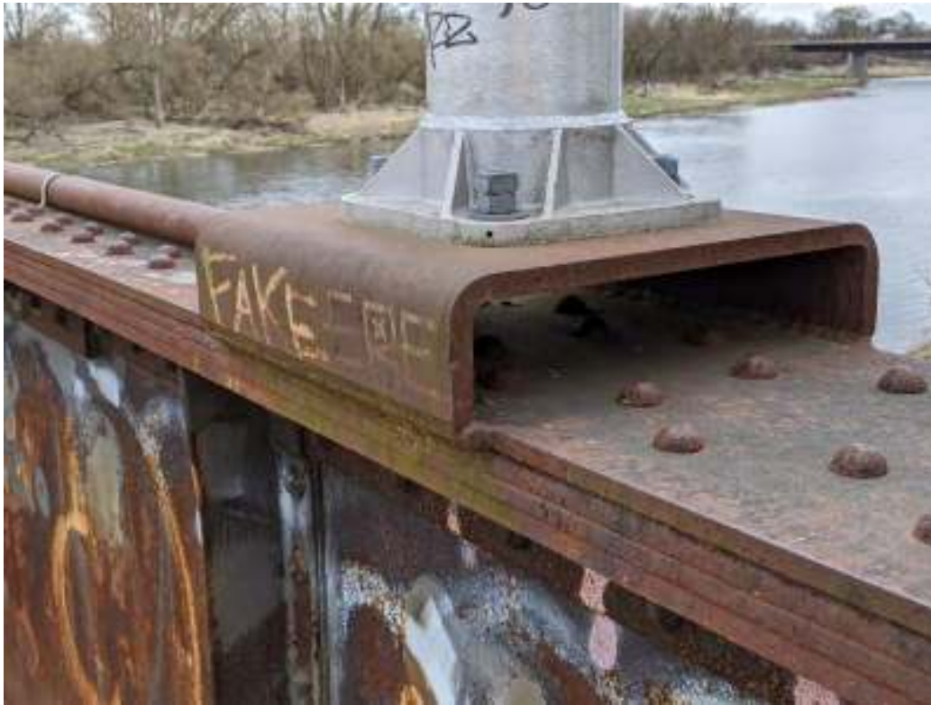
Figure 137: Conduit and aluminium light standard mounts on the top flange plate
