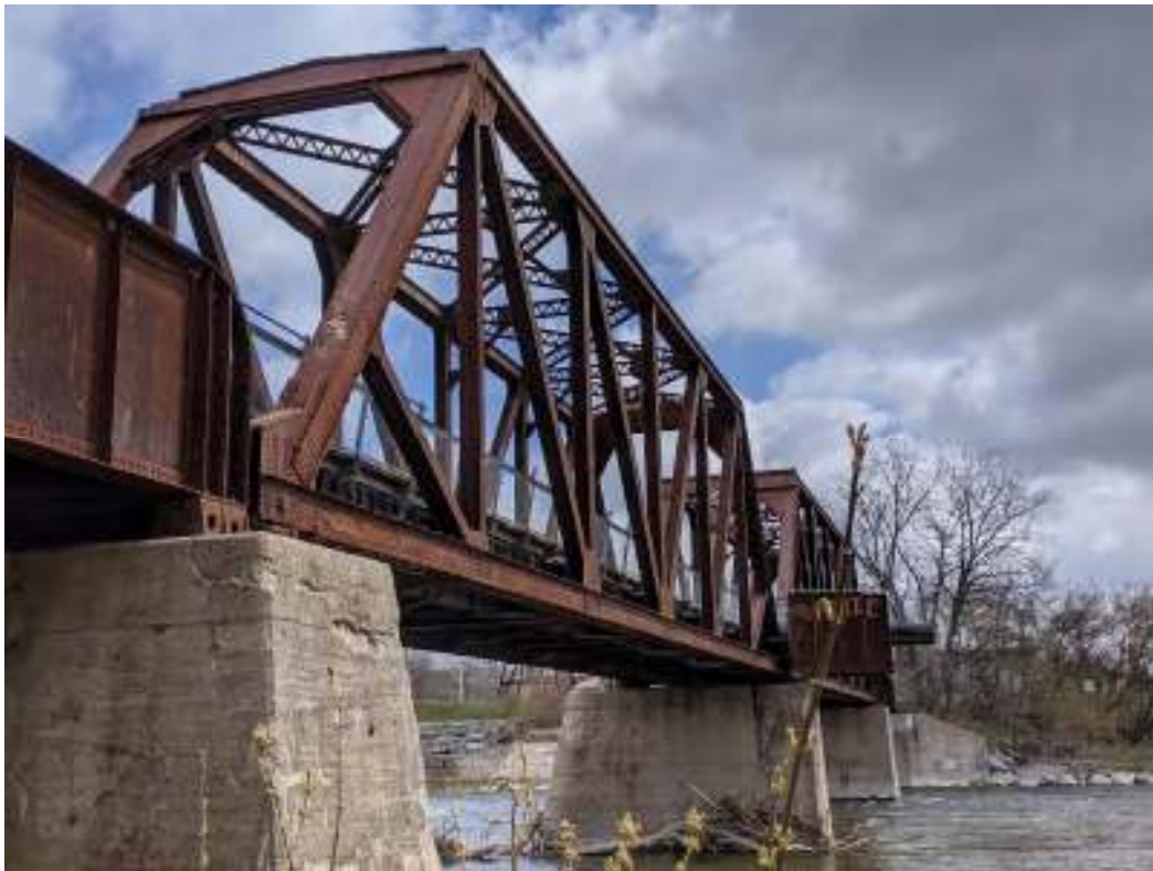
Figure 96: West and south sides of the west Pratt through truss span
