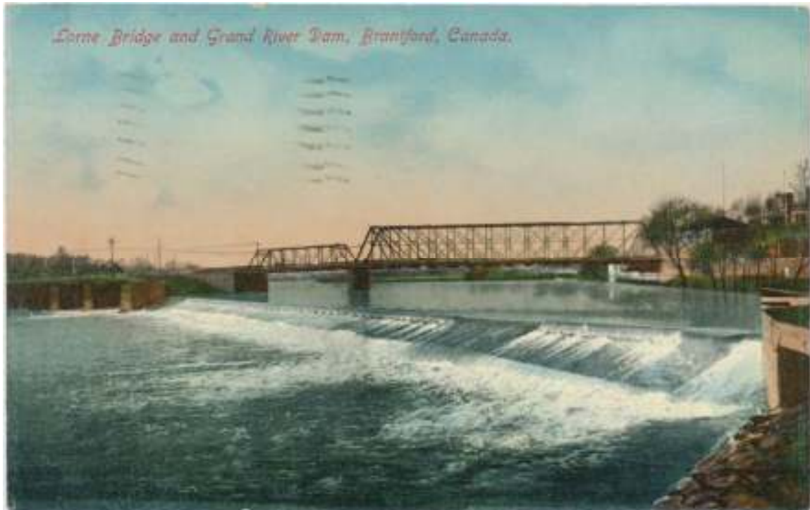
Figure 59: Postcard of the Lorne Bridge as seen from the south on the east bank (Brantford Public Library)
