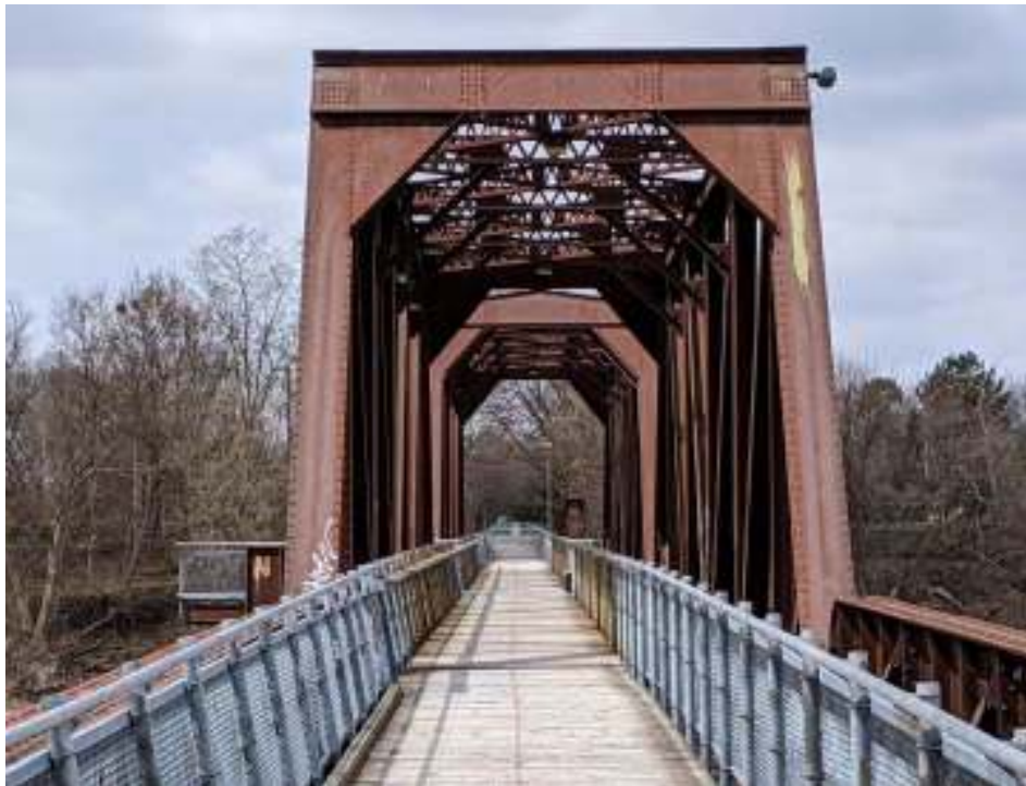
Figure 103: East portal of the east Pratt through truss span
