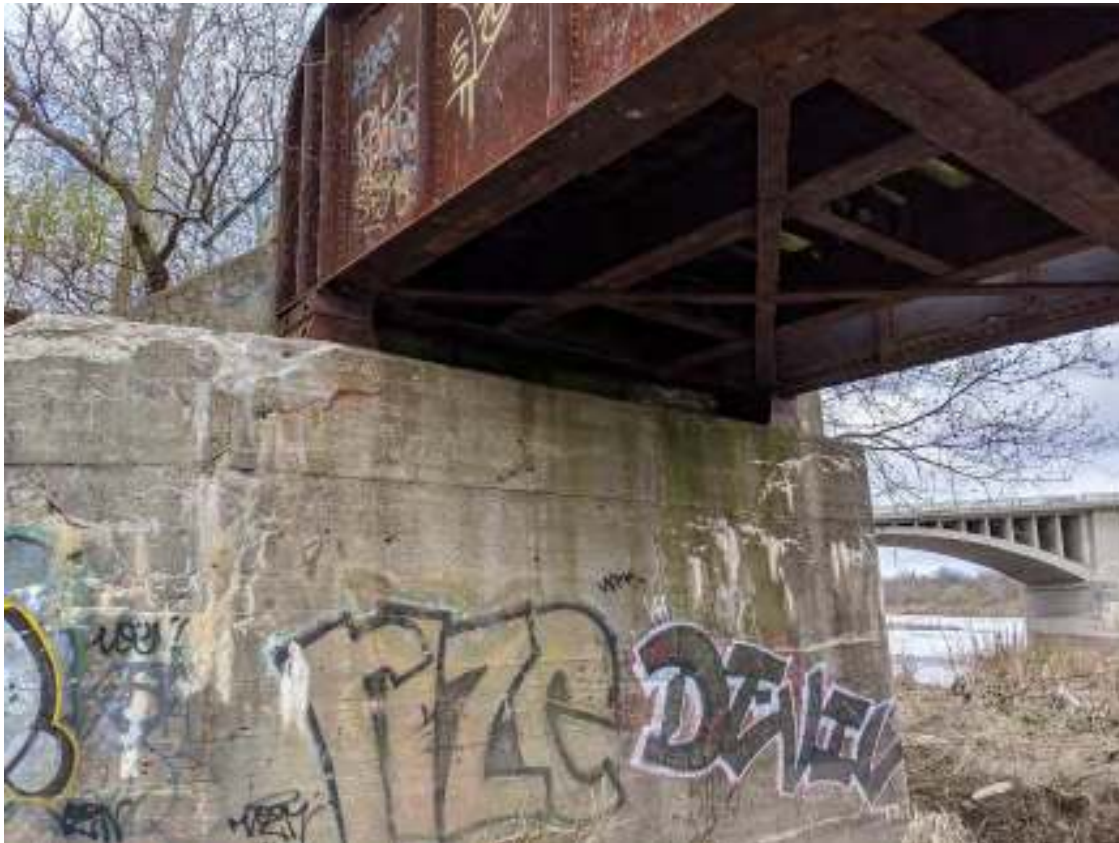
Figure 88: Front wall and ballast wall of the west abutment
