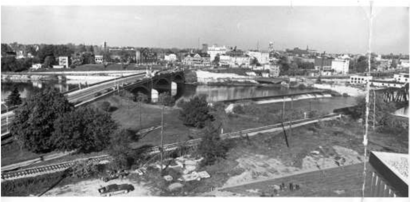
Figure 71: The Lorne Bridge in the 1970s (City of Brantford)
