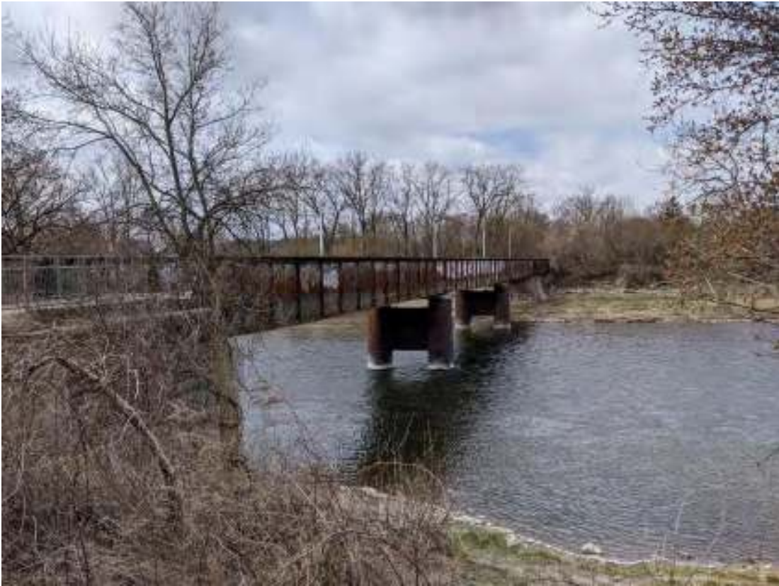
Figure 133: View facing west of the girder spans
