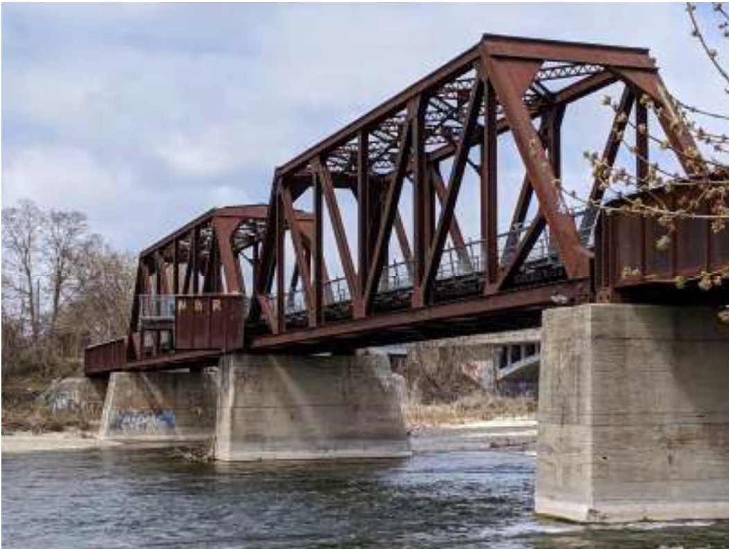
Figure 90: Downriver sides of the piers, facing northwest
