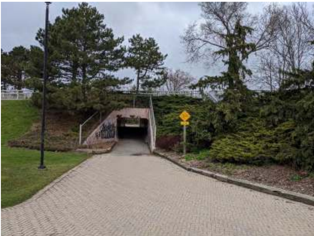
Figure 48: North headwall and wing walls of the concrete pedestrian underpass
