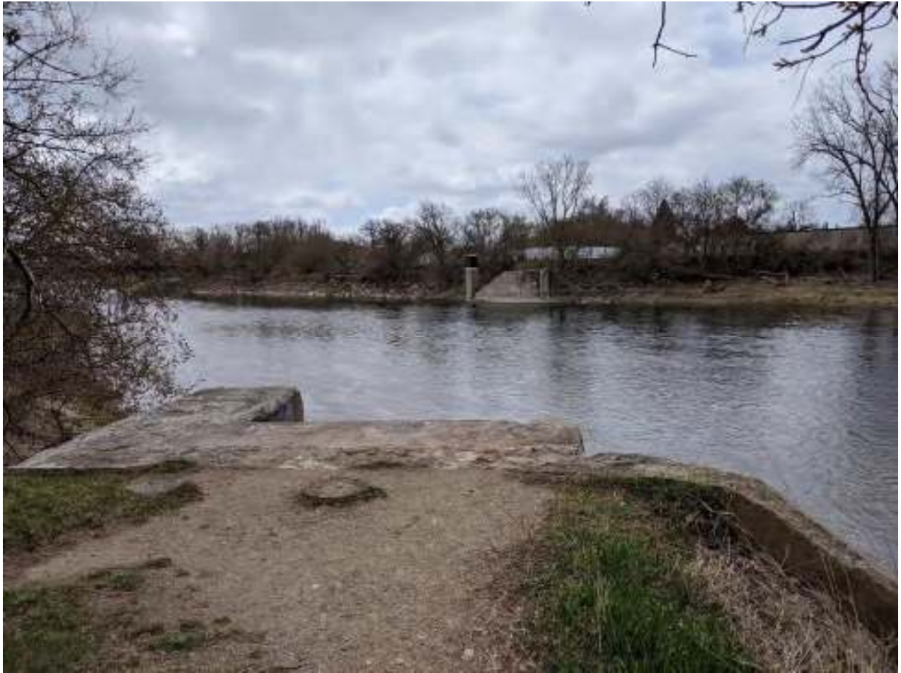
Figure 22: View facing southwest of the LE&N Railway Bridge abutments
