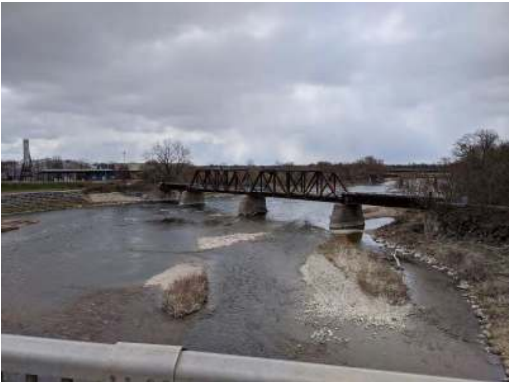
Figure 79: Setting of Brant's Crossing Bridge, facing south from the Lorne Bridge
