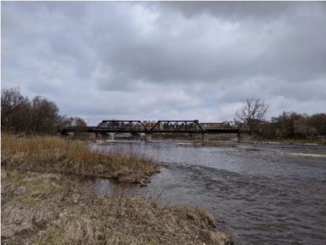
Figure 80: Setting of Brant's Crossing Bridge, facing north from the TH&B Crossing Bridge
