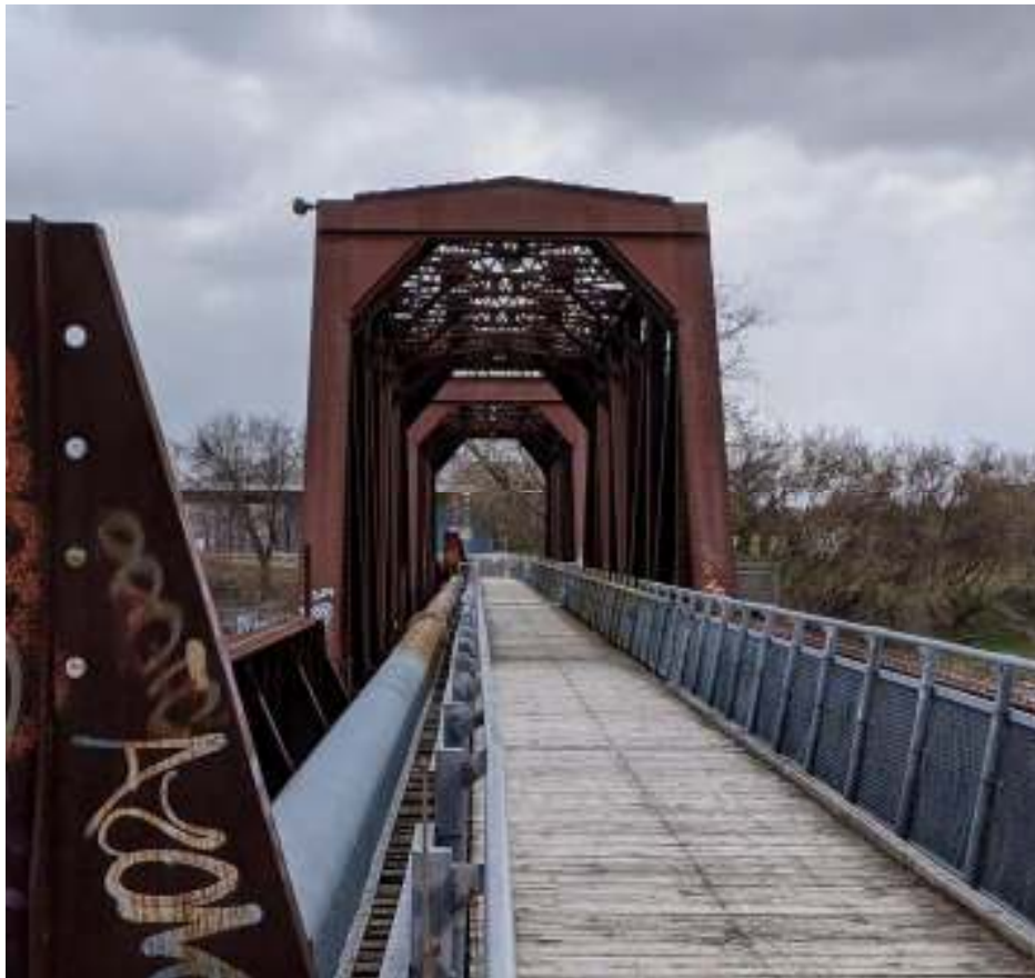
Figure 102: West portal of the west span
