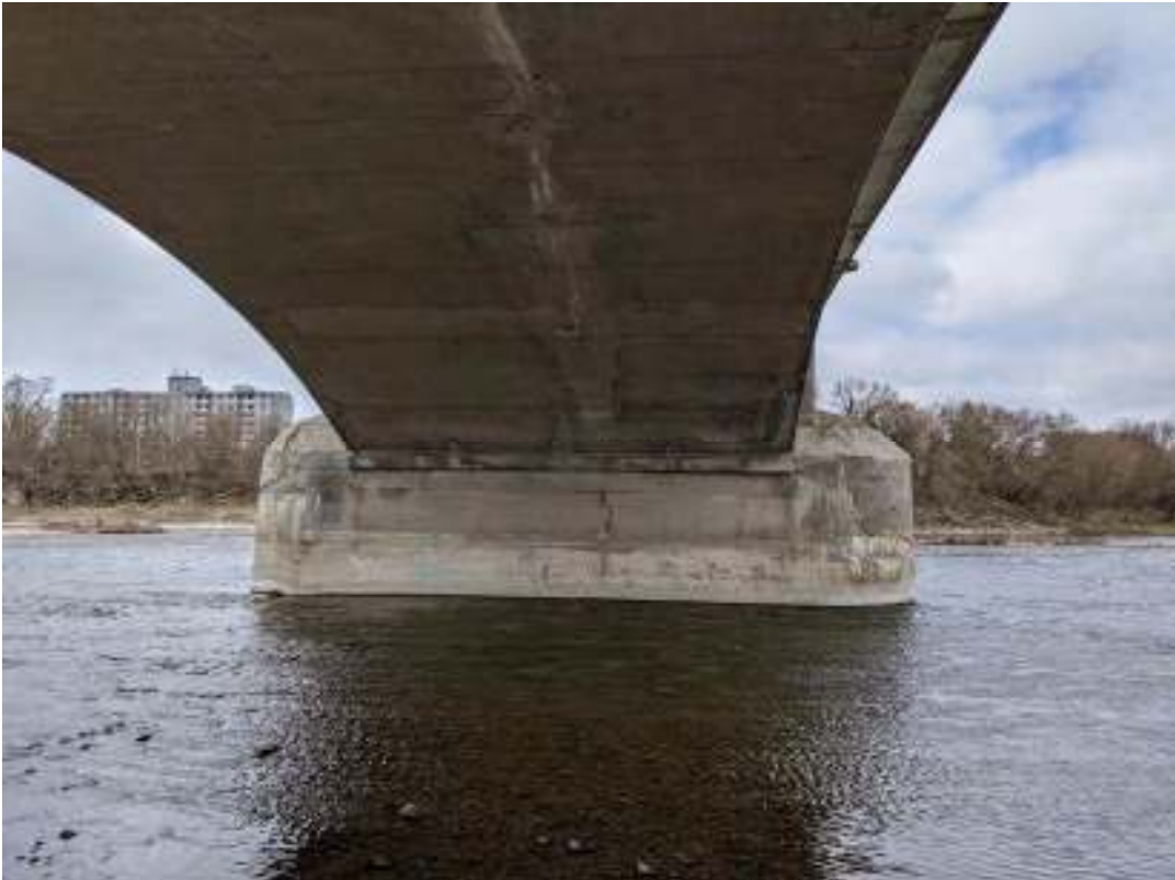
Figure 46: Spring of the arch at Pier No. 1
