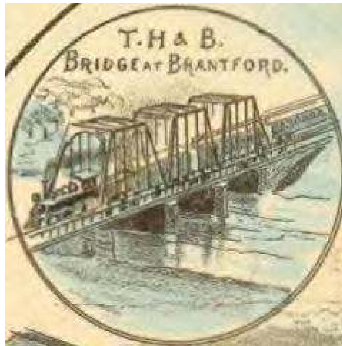
Figure 141: Inset on the 1892 Bird's Eye View of the TH&B Crossing Bridge
