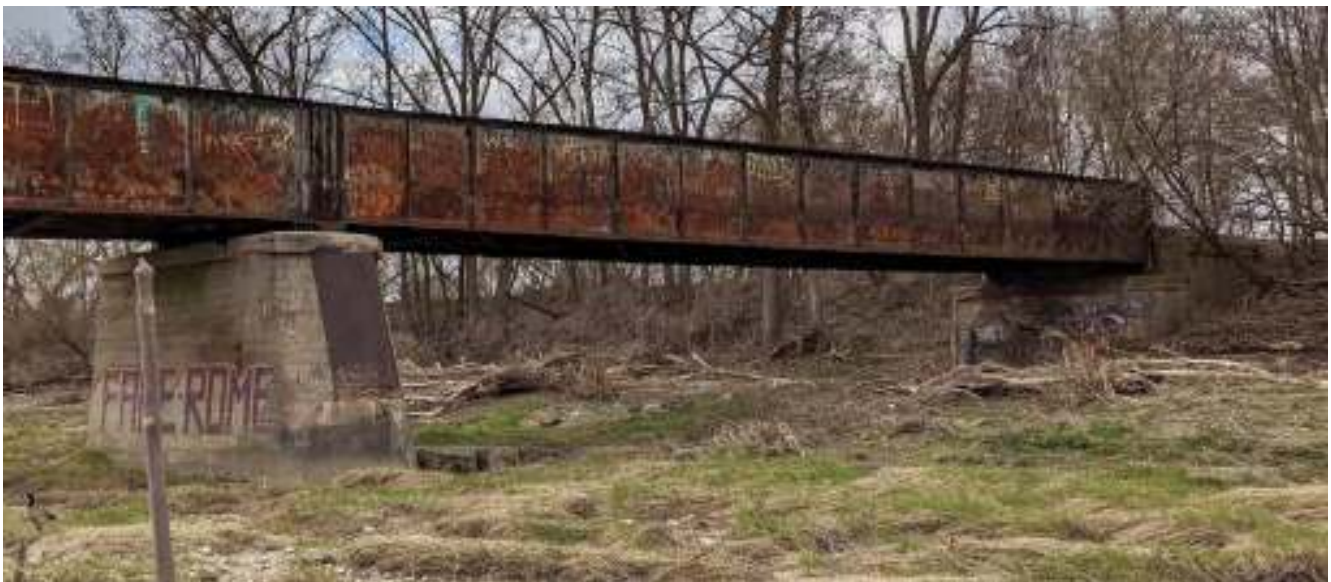
Figure 124: View facing southwest of the west abutment and pier
