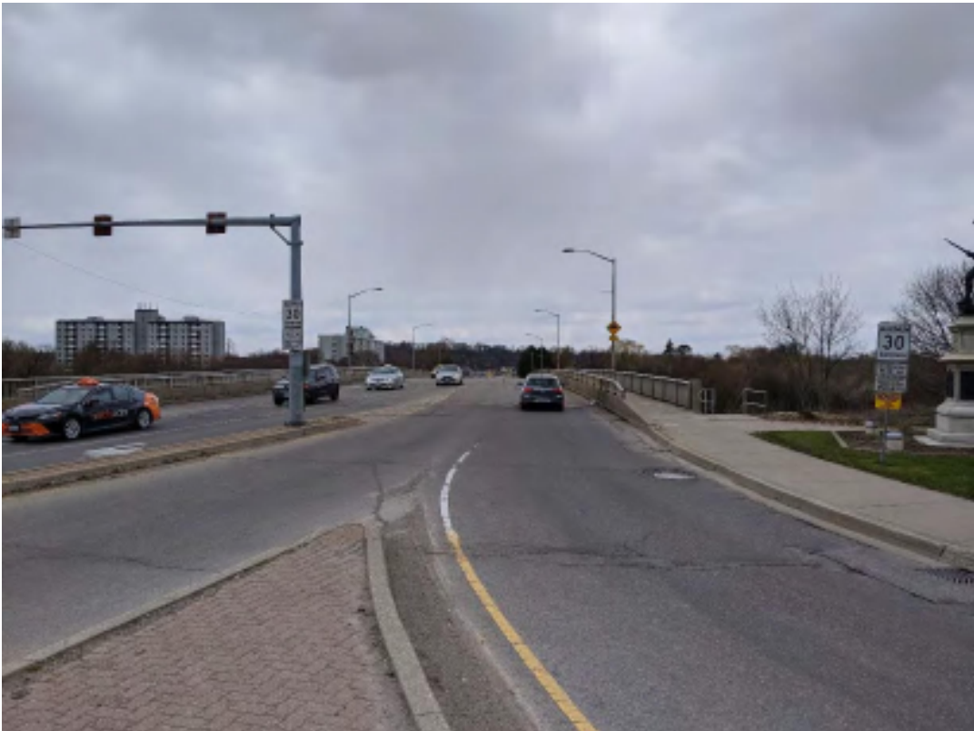
Figure 33: View facing west of the east approach
