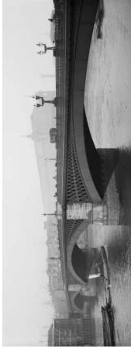
Figure 67: The Old Southwark Bridge spanning the Thames in London England, built in 1819 and replaced in 1921 (Historic England). Note the shallow arch spans, mouldings at the top of the sharp-nosed piers, and prominent parapet posts over the piers that match those of the Lorne Bridge (see Figure 68)
