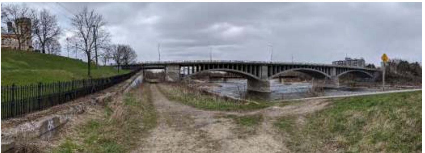
Figure 32: View of the Lorne Bridge facing south from the east bank.
