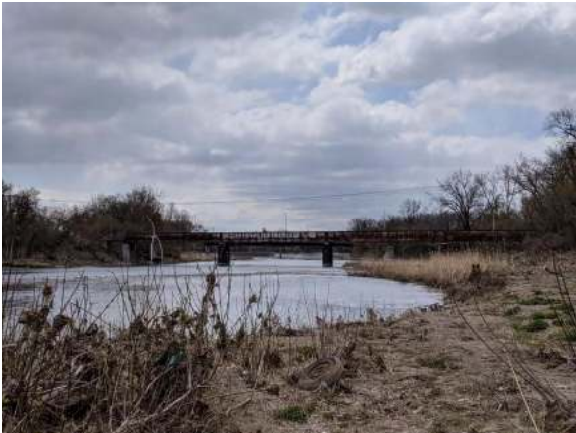
Figure 116: Setting of the TH&B Crossing Bridge, facing south from the west bank below Brant's Crossing Bridge
