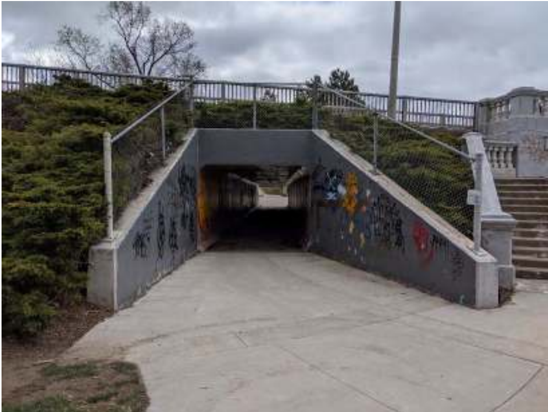
Figure 47: South headwall and wing walls of the concrete pedestrian underpass
