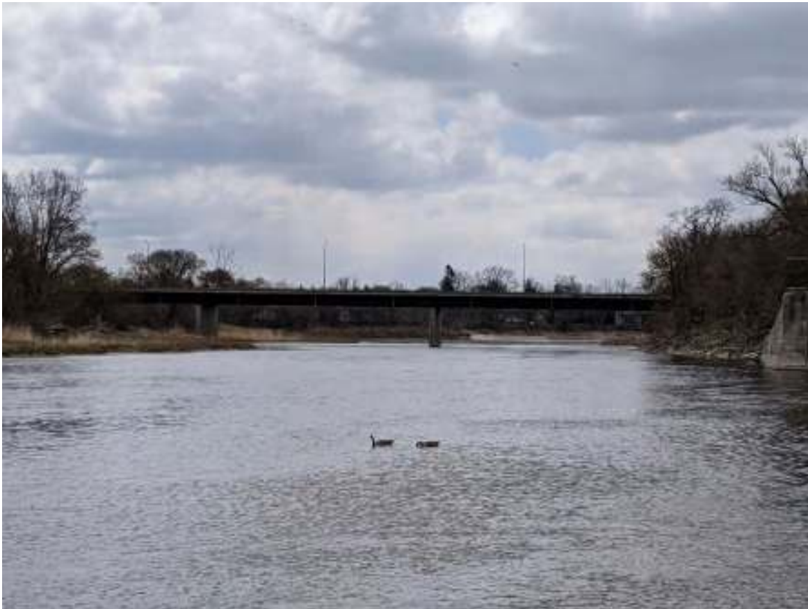
Figure 121: View facing south from the TH&B Crossing Bridge of the BSAR Bridge
