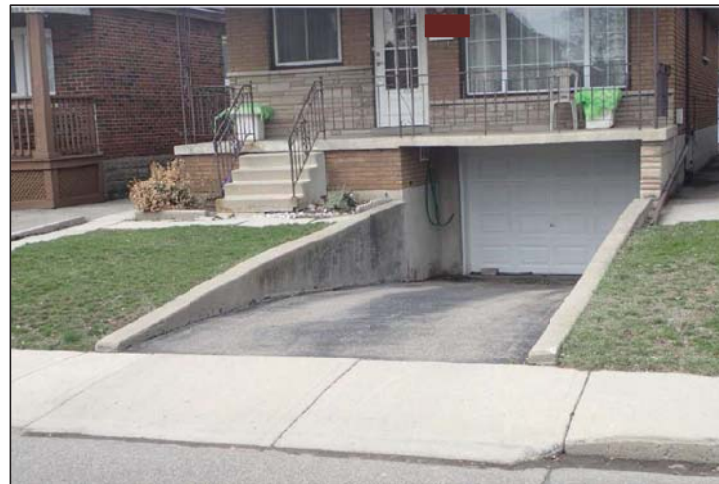
Homes with reverse slope driveways, without trench drainage in front of the garage, could be susceptible to overland flooding.
