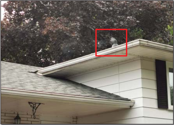
Smoke from plumbing vent, indicating potential cross-connection between sanitary lateral and storm sewer.
