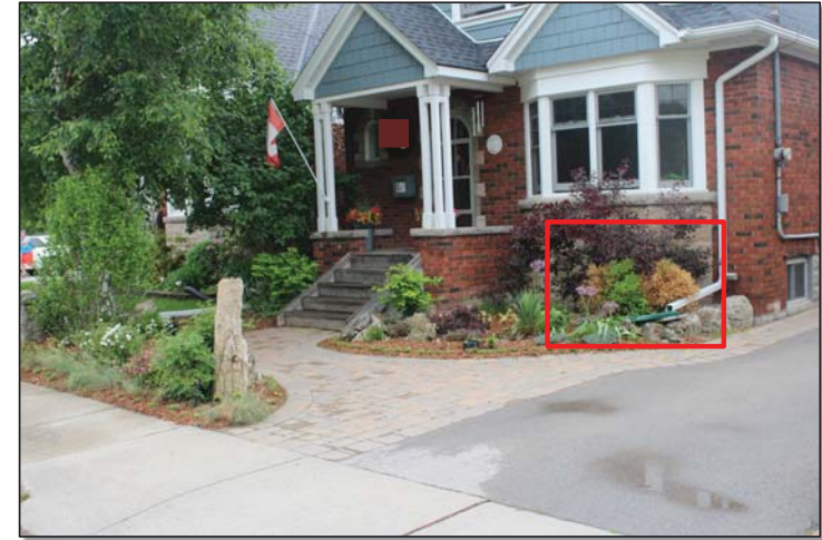
Disconnected downspouts (eavestroughs) direct flows to garden or lawn, which helps promote infiltration, reduce the amount of water entering the sewer system, and delays the time of water entering the sewer system.
