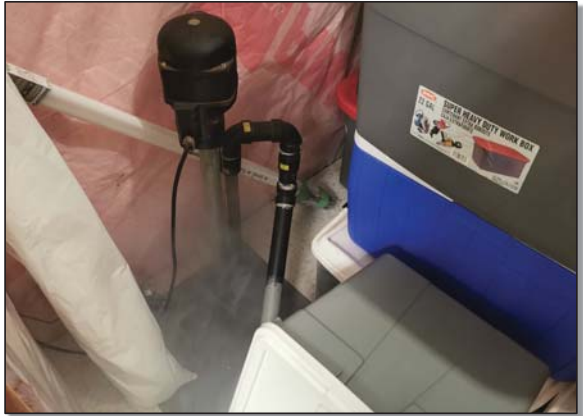
Basement sump pump was smoking, indicating direct connection to storm sewers on street.
