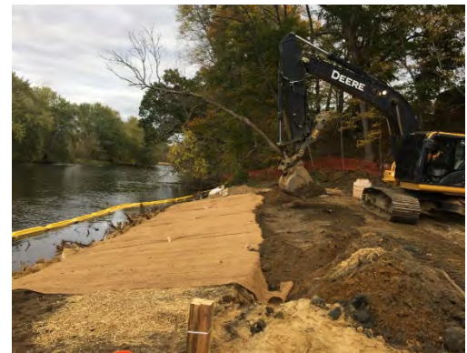
Shoreline Restoration Activities
