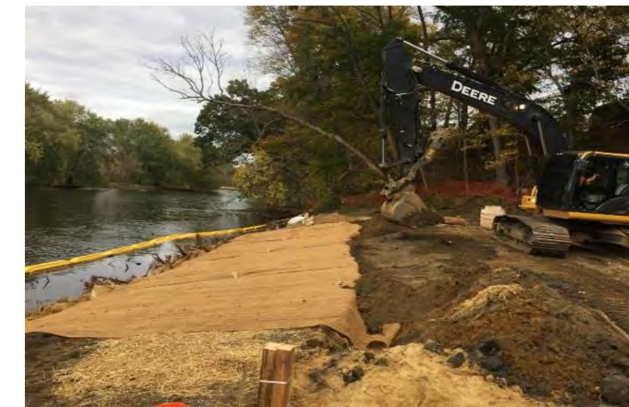
Shoreline Restoration Activities
