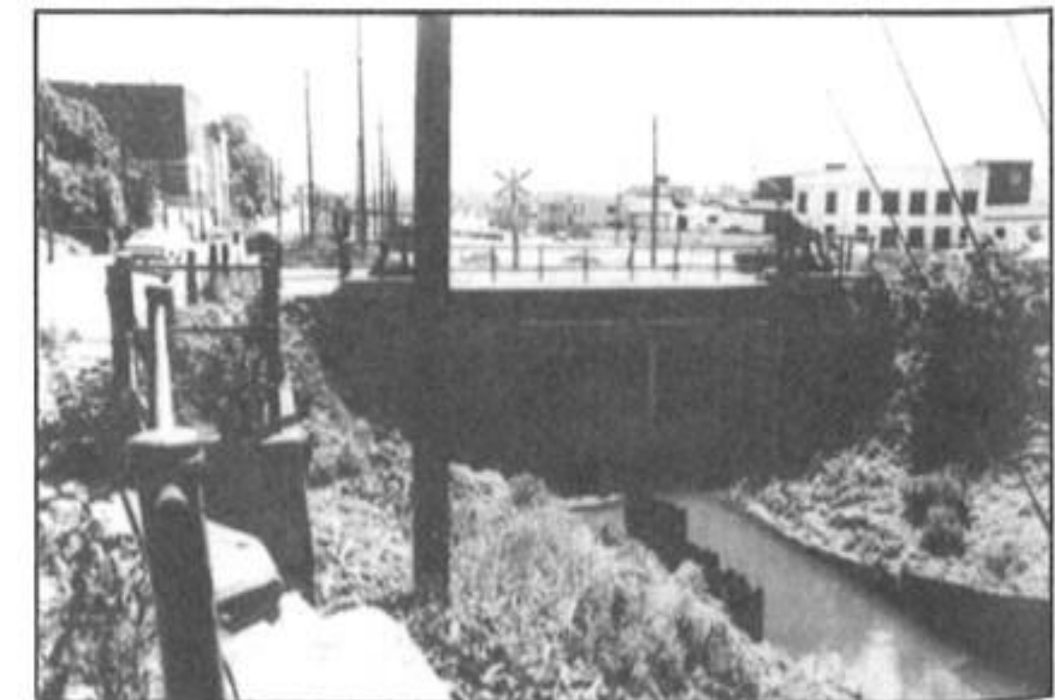
Remnant Of The Past – This is all that remains of the Grand River Navigation Canal which once flowed from the river, north of Greenwich Street, to Mohawk Lake. The sluice gate allows water to run through a buried pipeline to Mohawk Lake, whenever the river rises.
