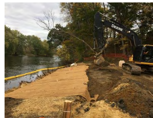
Shoreline Restoration Activities
