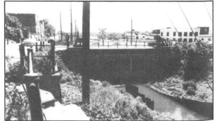
Remnant Of The Past – This is all that remains of the Grand River Navigation Canal which once flowed from the river, north of Greenwich Street, to Mohawk Lake. The sluice gate allows water to run through a buried pipeline to Mohawk Lake, whenever the river rises.
