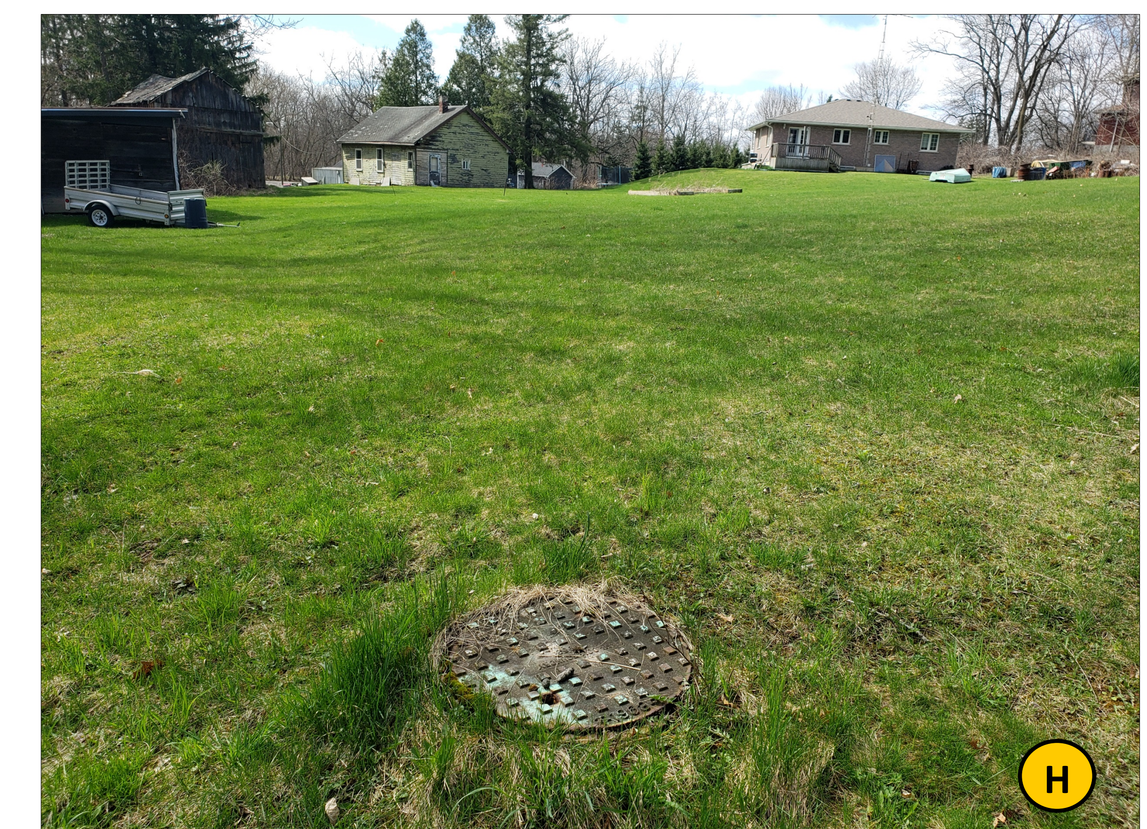
H. Sanitary manhole within private property, looking toward Peartree Court
