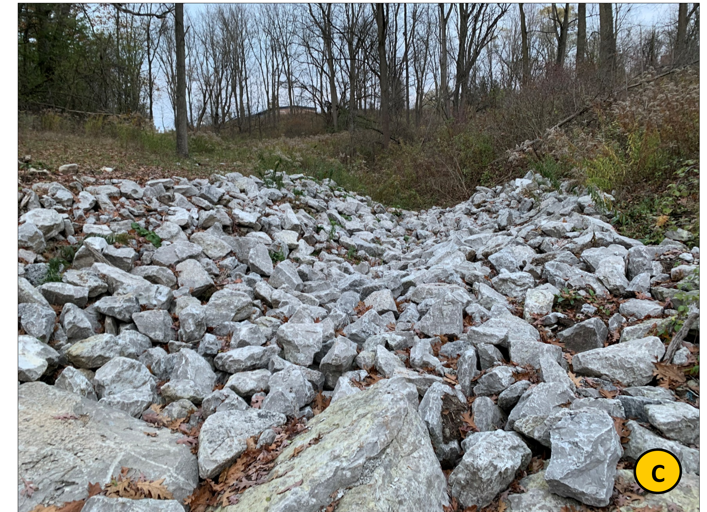
C. Previous emergency erosion protection for exposed sanitary sewer and manhole (2019)
