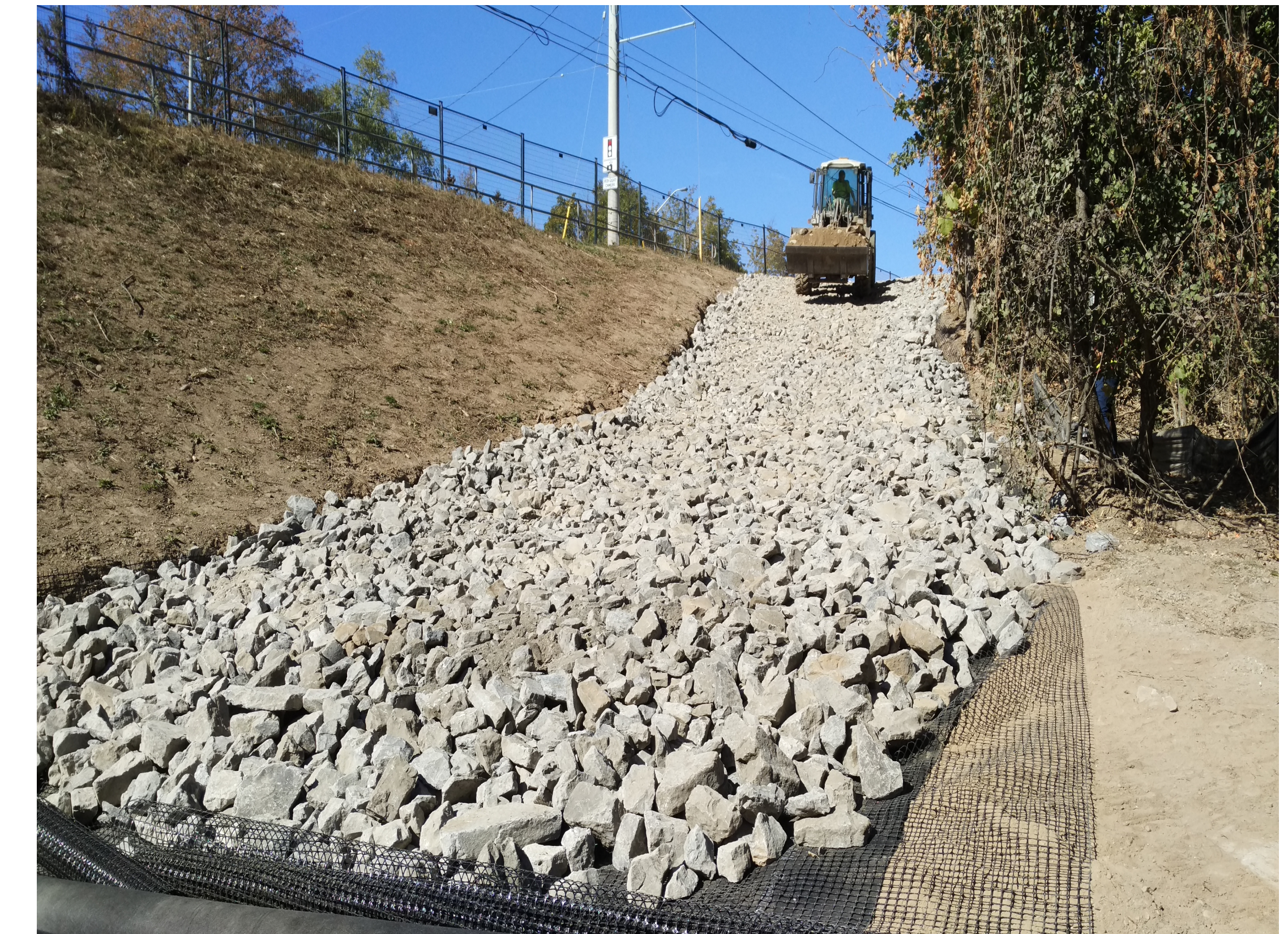
Rock Geogrid Access Road
