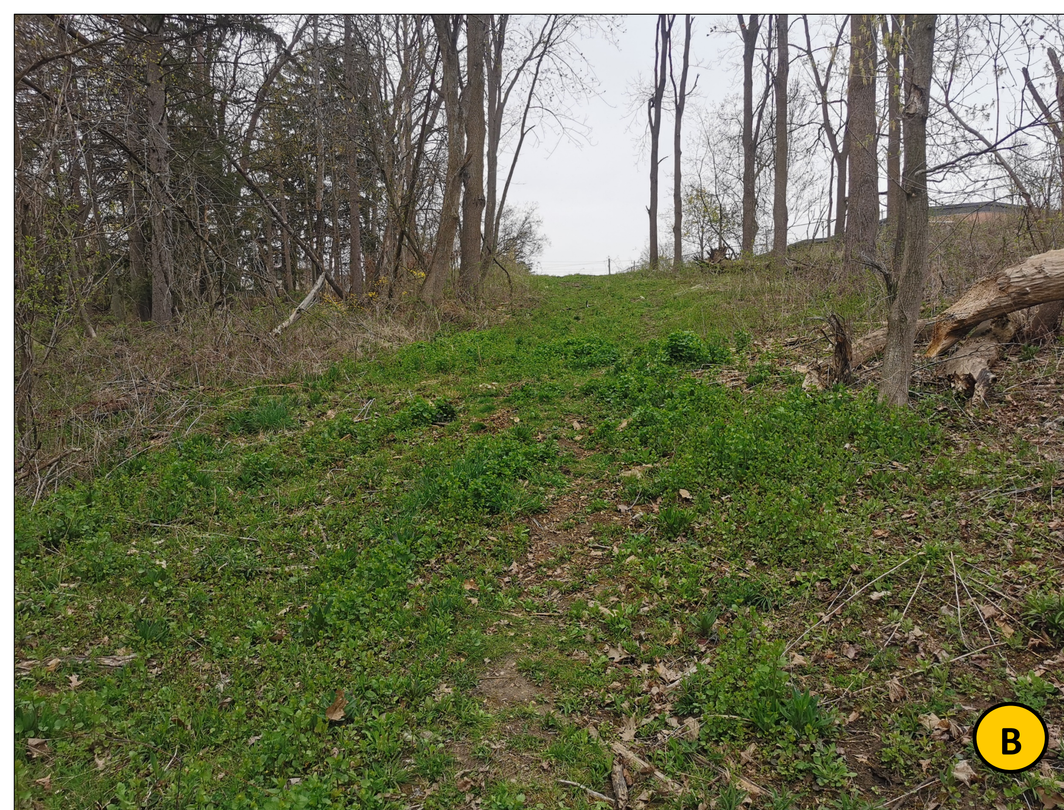
B. Steep slope along sanitary sewer easement from Glenwood Drive into valley
