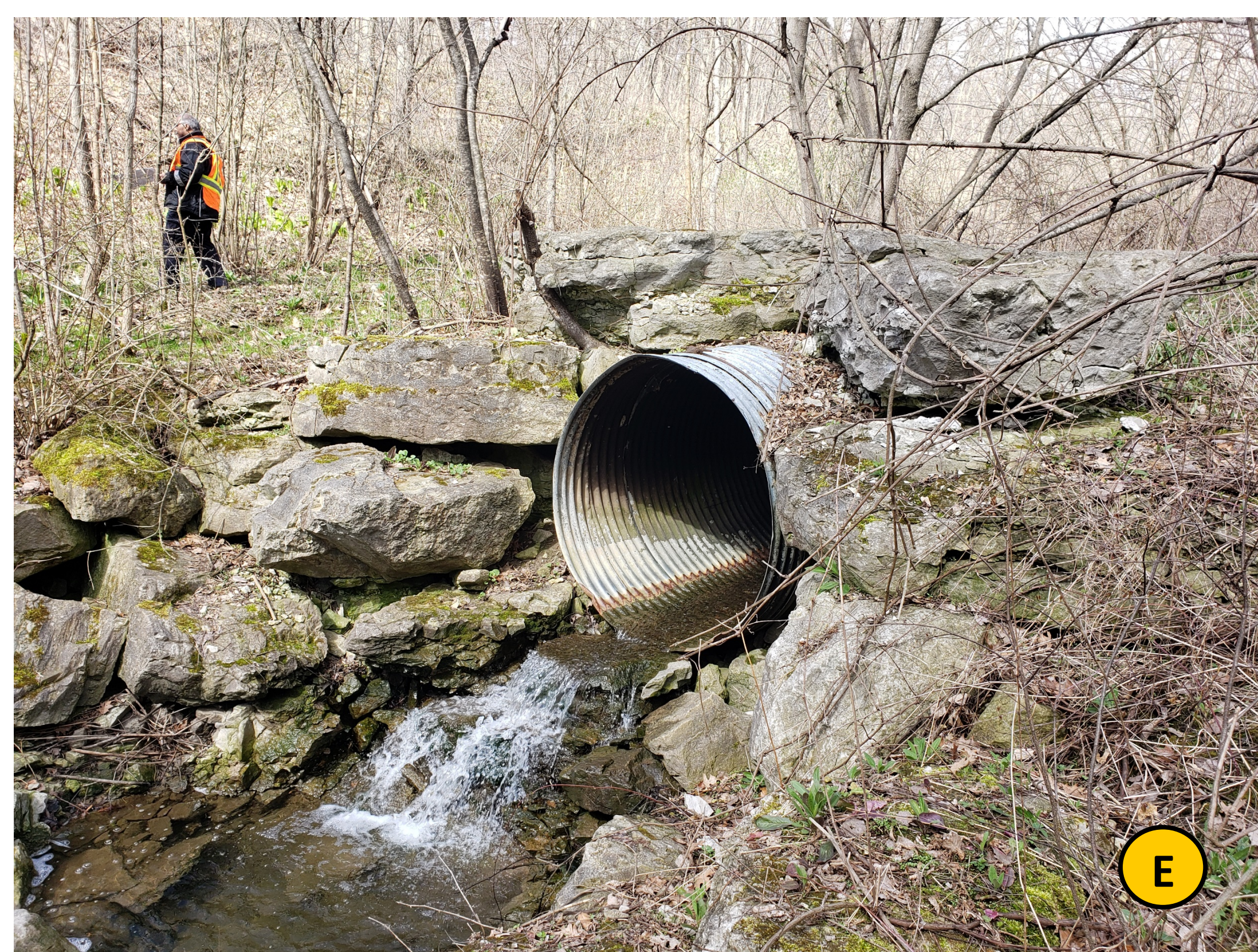
E. Existing CSP culvert over sanitary sewer crossing
