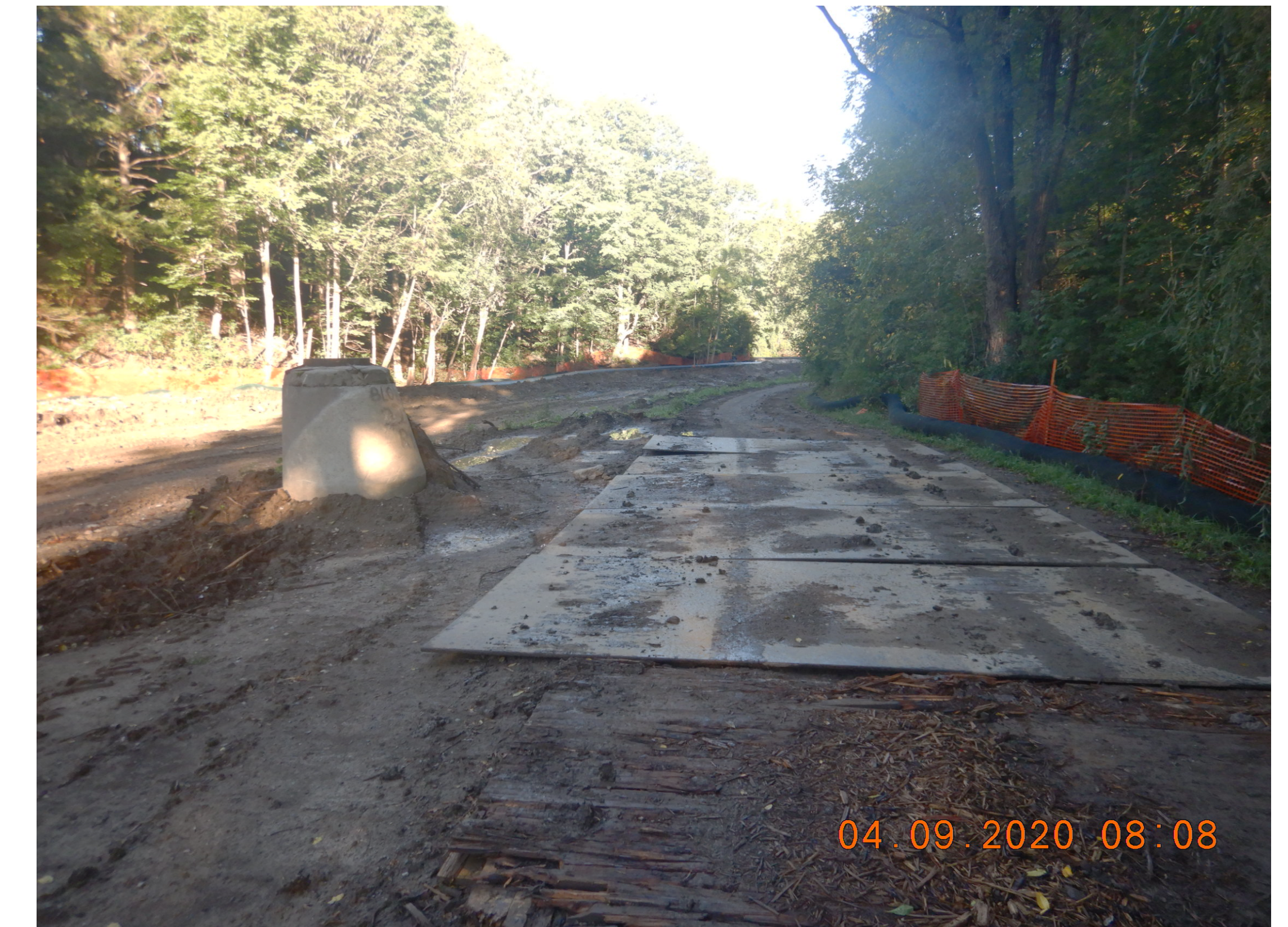
Temporary Steel Plates
