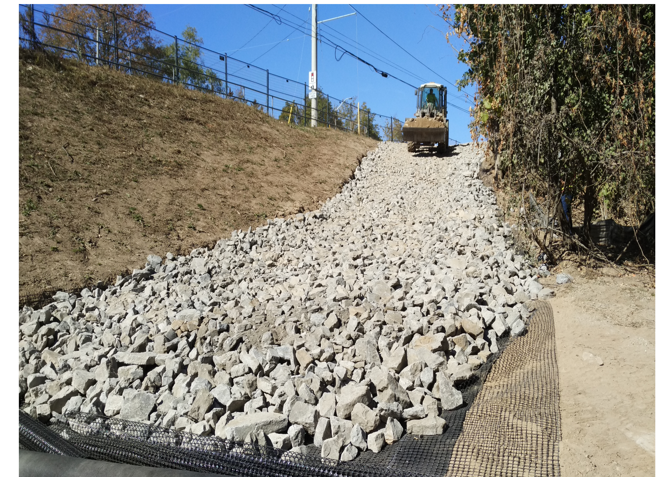
Rock Geogrid Access Road
