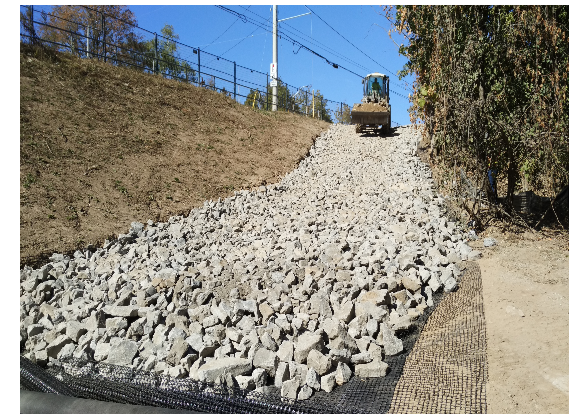
Rock Geogrid Access Road
