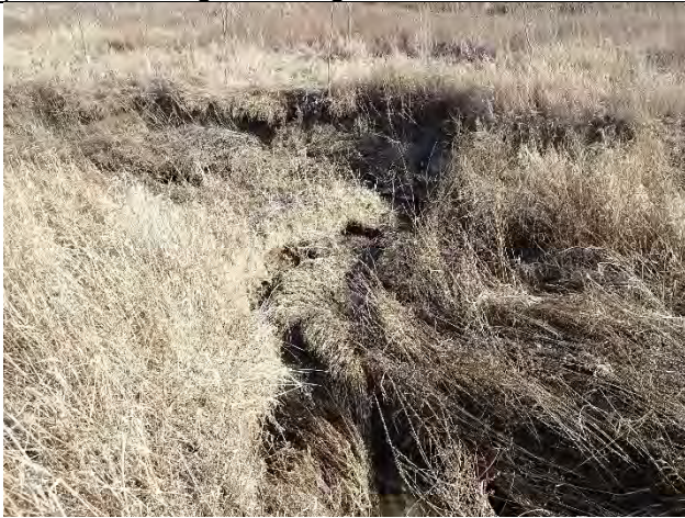
Photo 9: Erosion protection failure under pedestrian bridge crossing; undercut bank.
