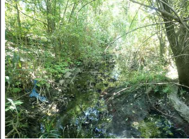
Reach 3: Vegetation and root masses have established over the cable concrete.
