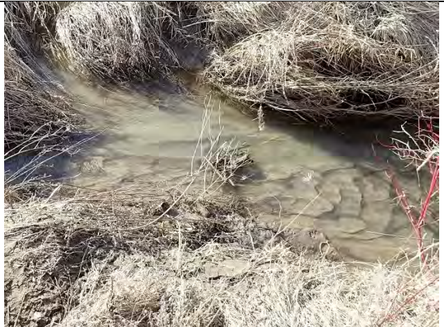
Photo 10: Channel bank erosion and slumped material into channel.
