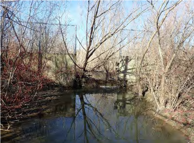
Photo 5: Downstream view of concrete weir.
