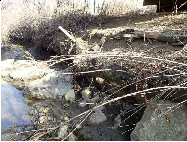
Photo 9: Erosion protection failure under pedestrian bridge crossing; undercut bank.
