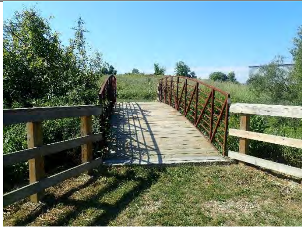
View of pedestrian crossing bridge over watercourse.
