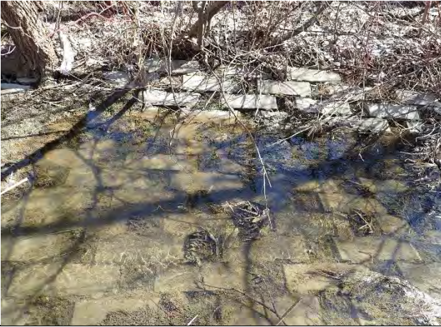
Photo 3: Cable concrete lining on channel bed.
