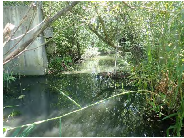
Reach 3: View downstream as water flows over concrete weir.
