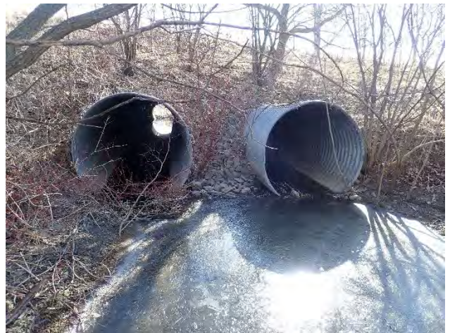
Photo 8: Double culvert at SWM facility embankment.
