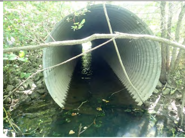
Reach 2: View through large culvert present at boundary between Reach 2 and 3.
