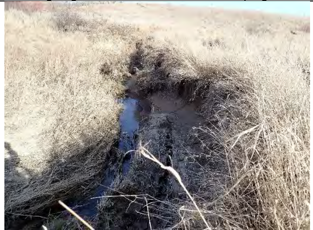
Photo 6: Bank erosion and slumped bank material into the channel.
