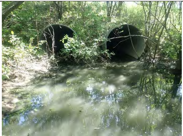
View of two corrugated steel culverts present within the watercourse.
