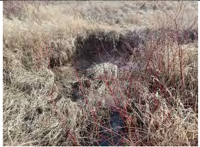
Photo 10: Channel bank erosion and slumped material into channel.
