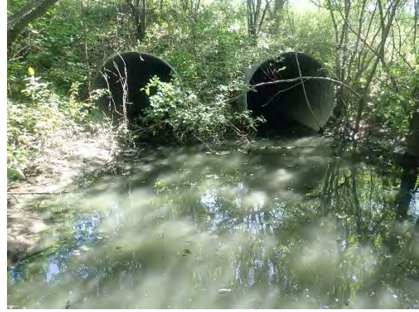
Reach 3: View of large twin culverts at Reach 2 and 3 boundary.
