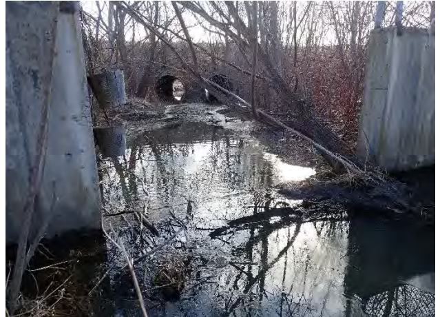
Photo 6: Downstream view of SWM facility embankment from concrete weir.
