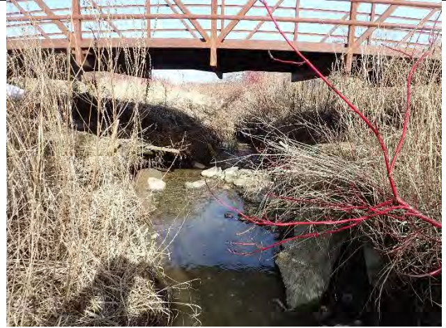
Photo 8: Pedestrian bridge crossing.
