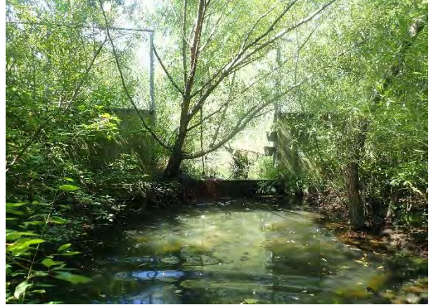
View of concrete weir present in watercourse in proximity to SWMF.
